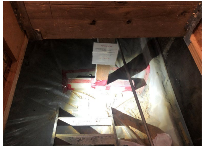
Photo 6. Sign regarding vapor barrier posted just inside crawlspace access point.
