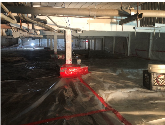
Photo 3. Bamboo Panda crawlspace vapor barrier repair. Looking north.
