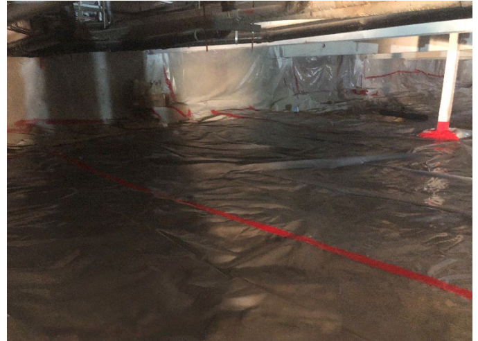
Photo 4. Bamboo Panda crawlspace vapor barrier repair. Looking west.
