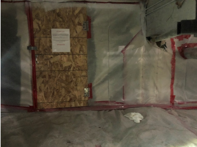
Photo 7. Sign regarding vapor barrier posted on door separating the F&H Fitness and Bamboo Panda crawlspaces.
