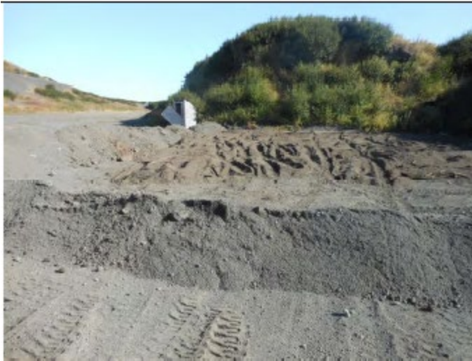
Figure 5. Landfarm in 2015 directly after construction (TPECI 2015)
