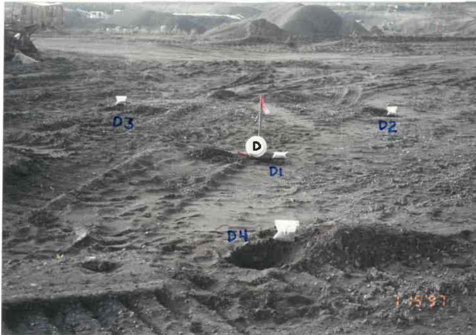
Looking northwest at area D - test holes D1, D2, D3 and D4 note: Active pit area is in the background
