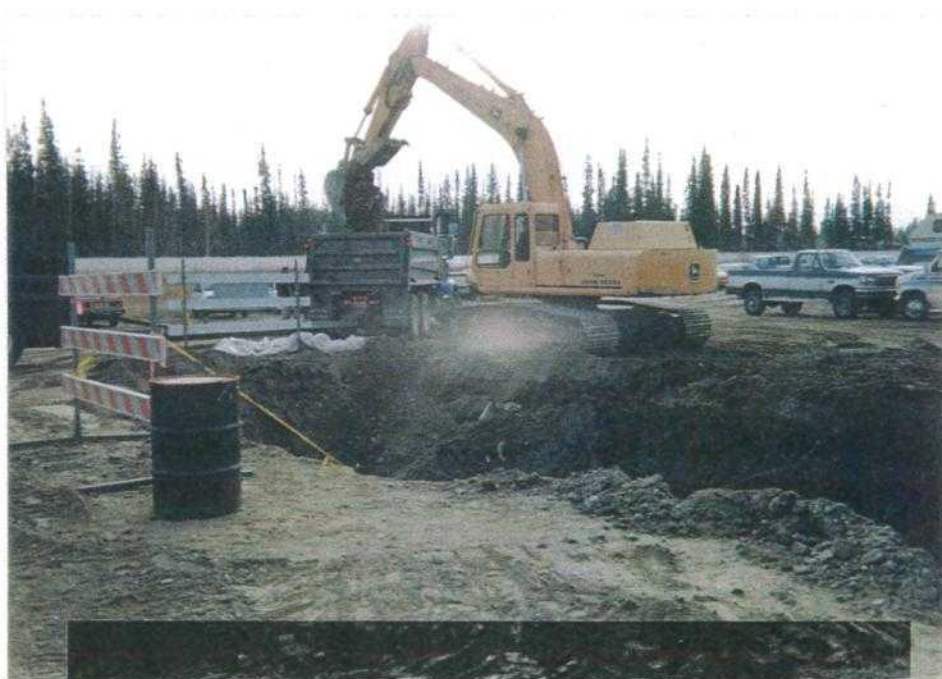
Photo 8: Impacted soils were loaded directly into trucks for disposal hauling.
