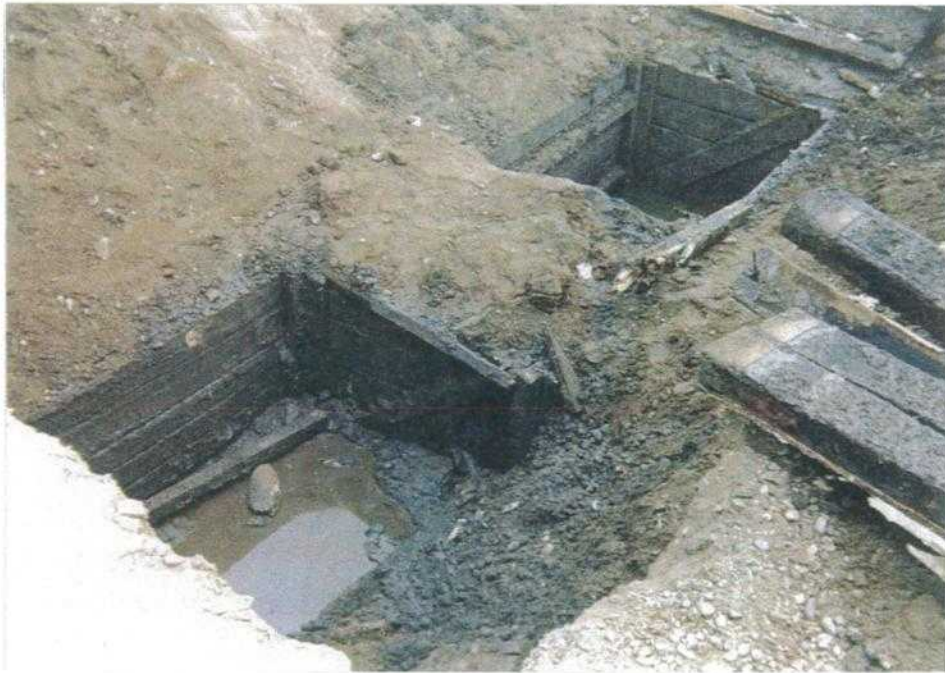
Photo 3: Two septic cribs were encountered south of the septic tank area. Note stained soils at photo bottom center.
