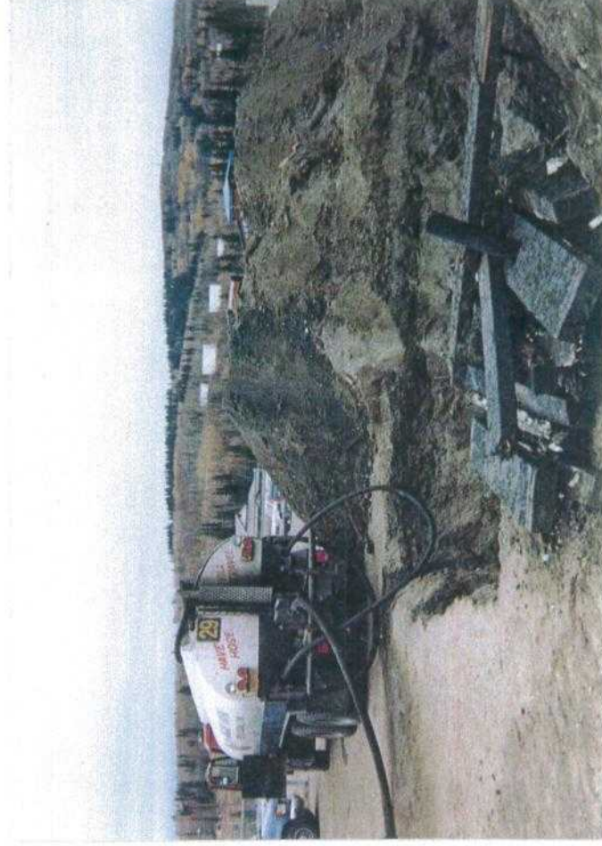
Photo 2: Pumping of septic tank.
