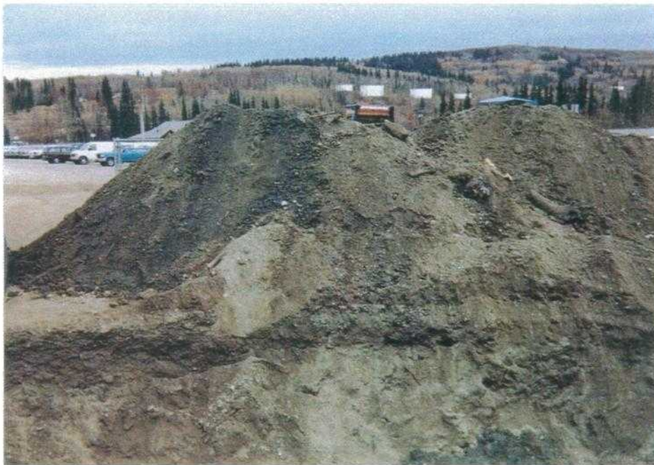
Photo 4: Excavated soils were temporarily stockpiled on site prior to disposal hauling.
