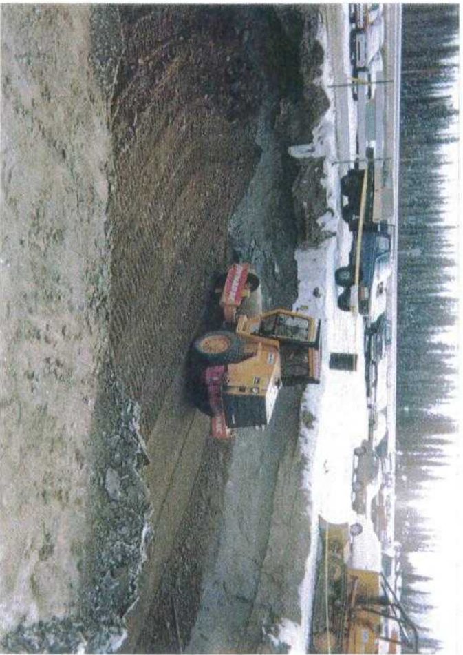
Photo 10: View of compaction during site backfill.
