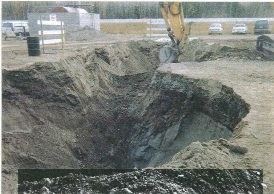
Photo 7: View of excavation during the removal of impacted soils. Note the diked aboveground storage tank at top left.
