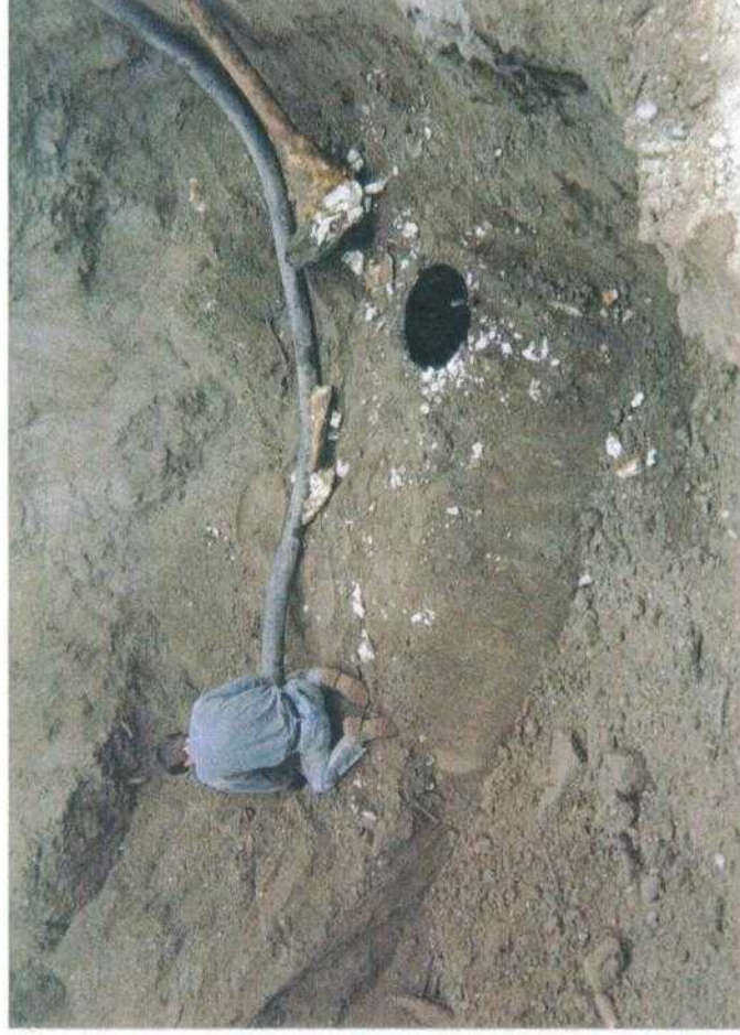
Photo 1: View of in-place septic tank associated with the former injection well.
