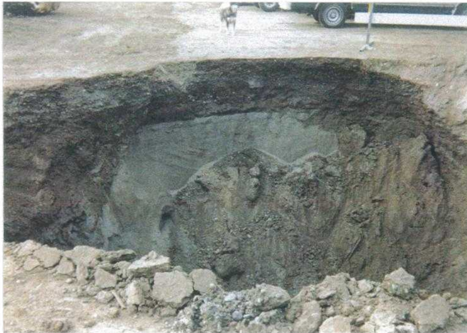
Photo 5: View of southwestern corner of the excavated crib area showing variable soil conditions.
