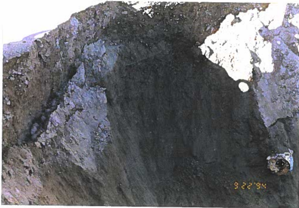
Photo 10: View of northwest corner of the excavation.
