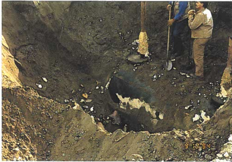
Photo 7: Septic tank during removal.
