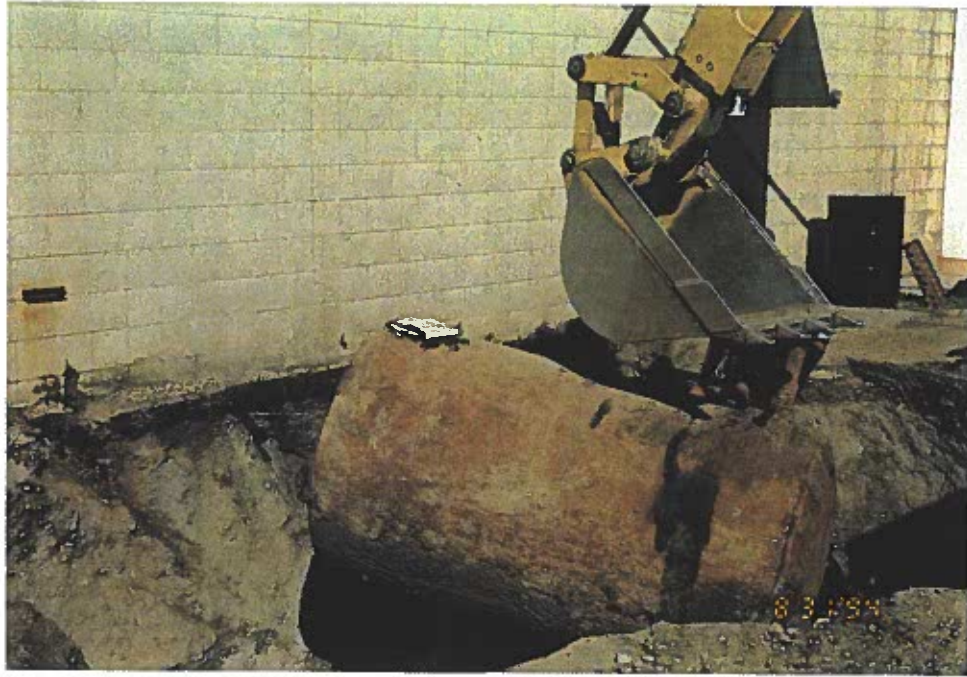
Photo 3: UST No. 1 during removal.
