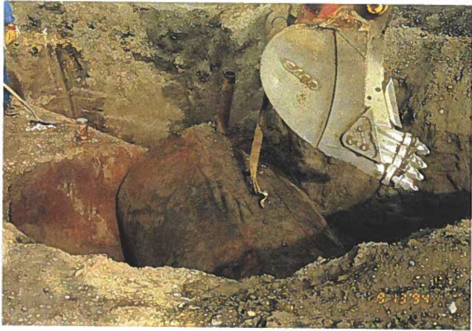
Photo 3: UST No. 3 during removal.
