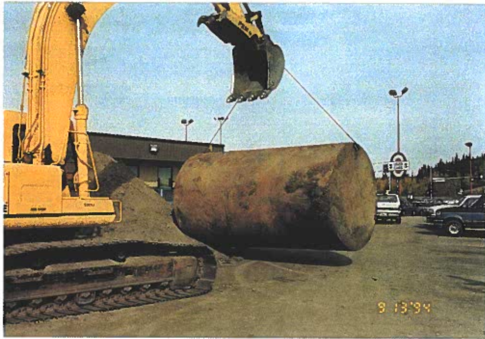
Photo 5: UST No. 4 during removal.
