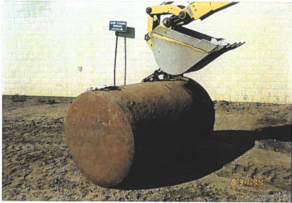
Photo 4: General condition of UST No. 1.
