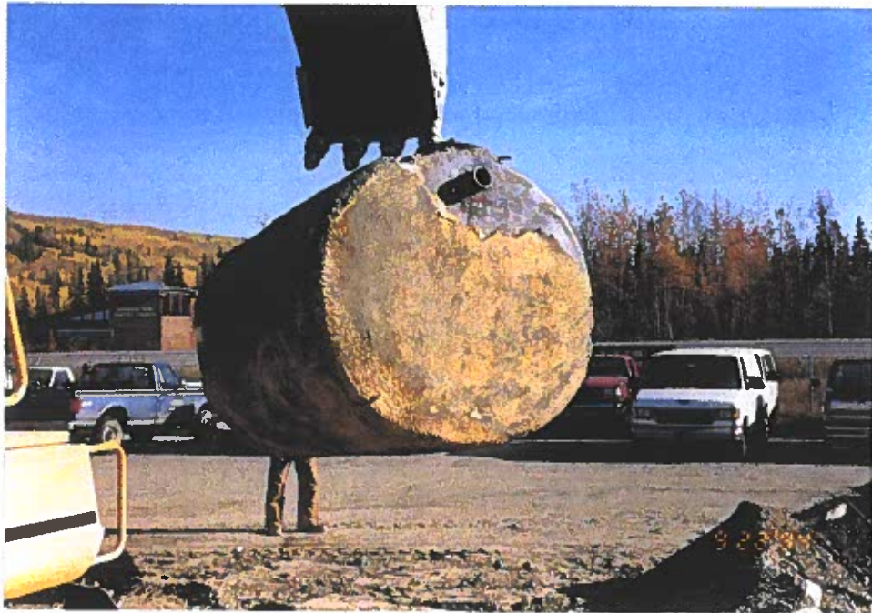
Photo 8: Septic tank during removal.
