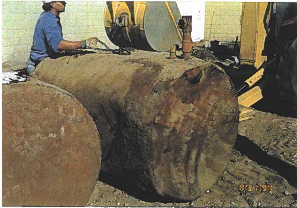
Photo 7: General condition of UST No. 2.
