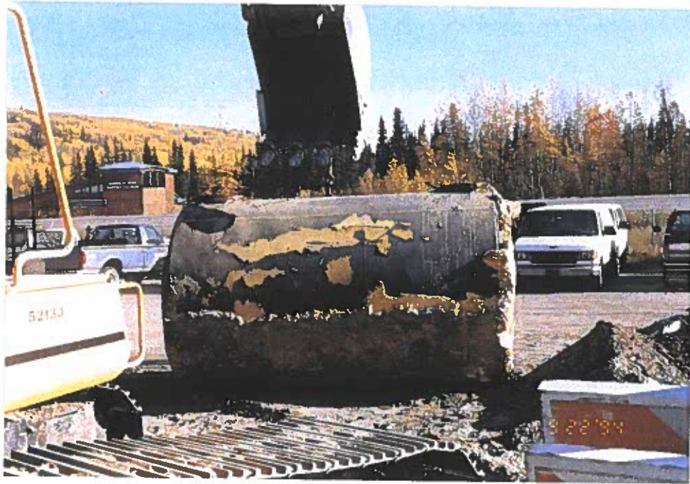
Photo 9: General condition of removed septic tank.
