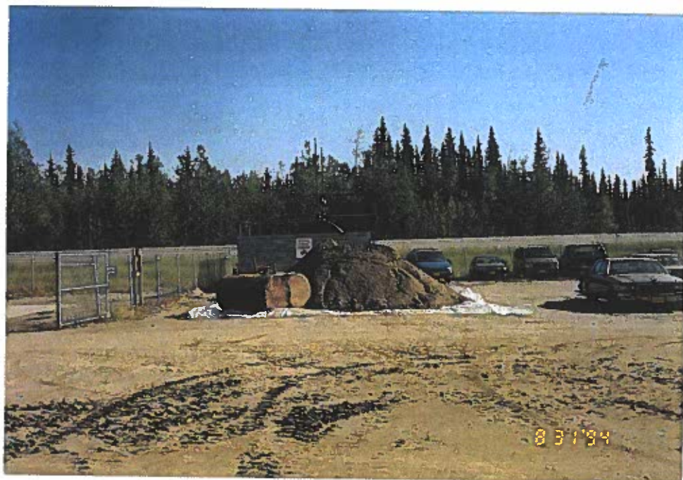
Photo 10: Impacted soils were stored on 10-mil reinforced polyethylene liner pending sample laboratory analysis. Note the recently installed aboveground storage tank system in background.
