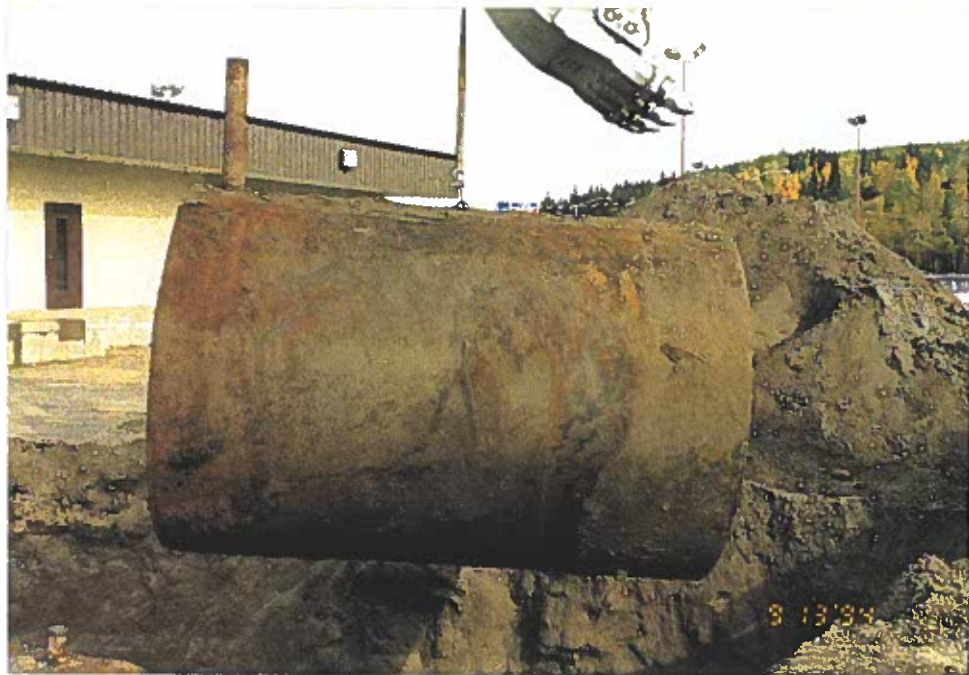
Photo 4: General condition of UST No. 3.
