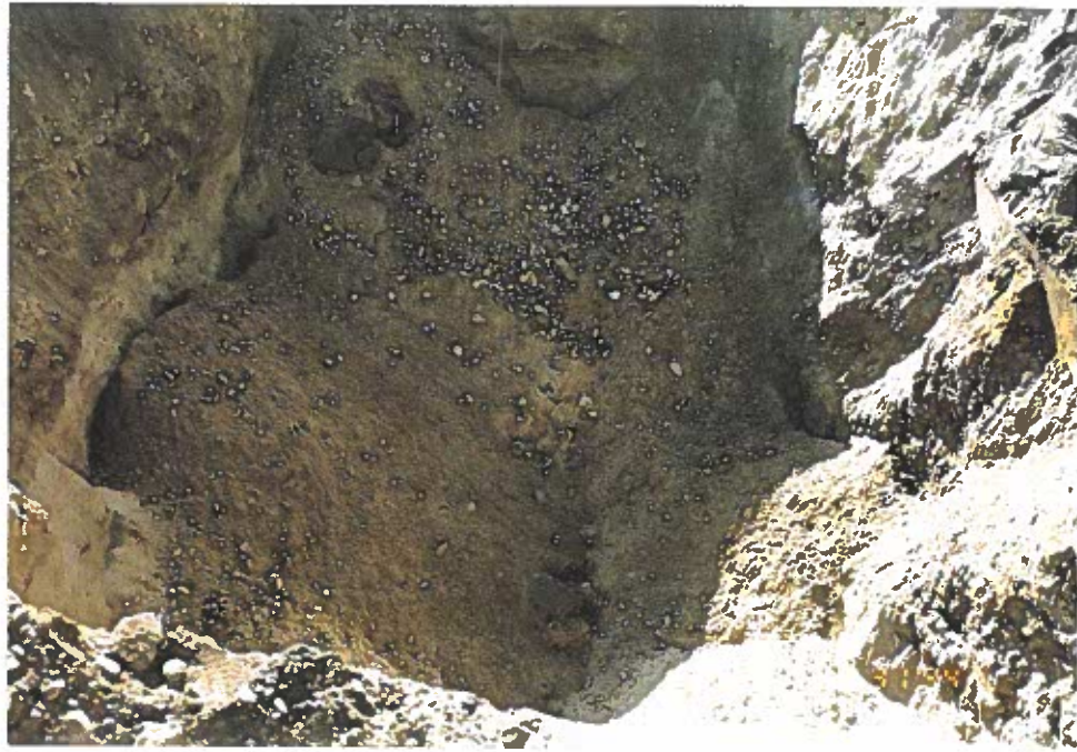
Photo 9: View of excavation base during the removal of impacted soils.
