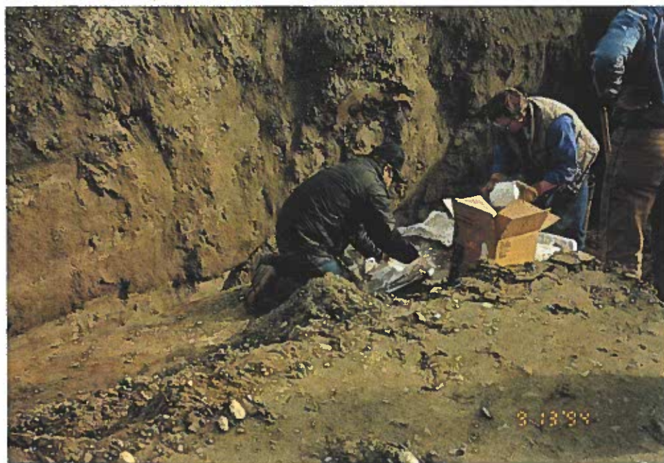
Photo 2: The tanks were purged with air to reduce the level of explosive vapors inside the tanks and then were inerted with dry ice.
