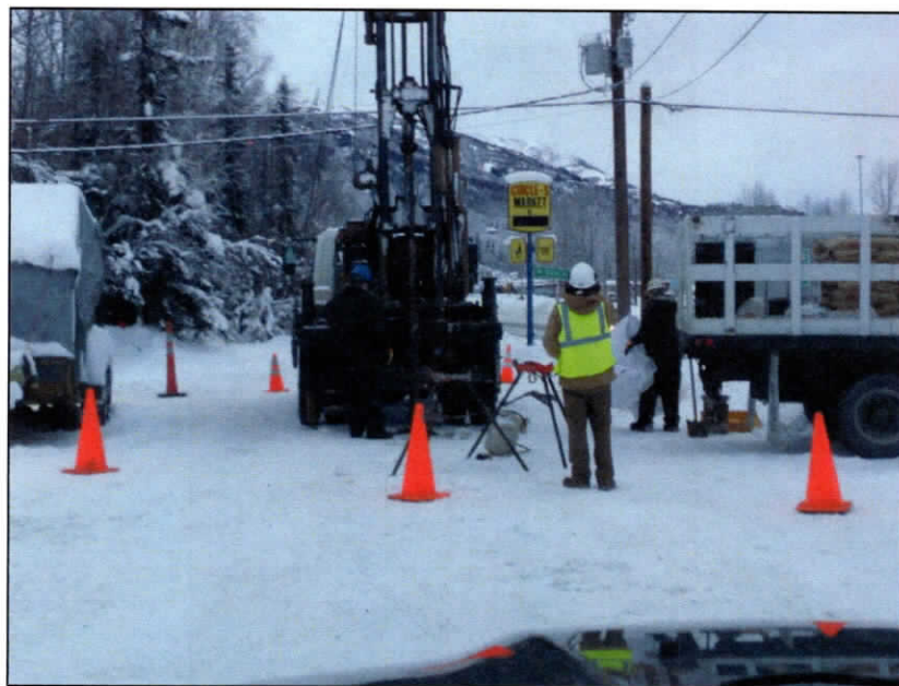
PHOTOGRAPH 10: DRILL RIG SET UP AT BOREHOLE 1
