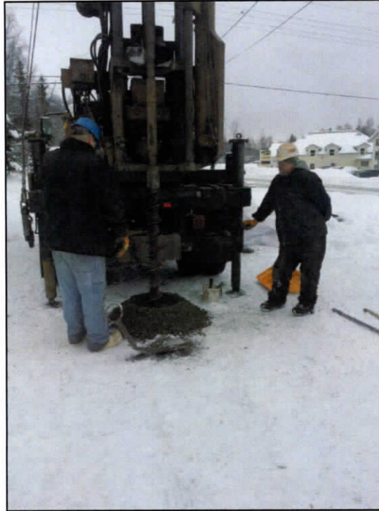
PHOTOGRAPH 11: DRILLRIG SET UP AT BOREHOLE 3
