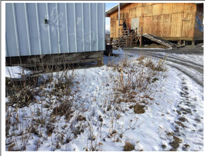
Photograph 5: Looking northwest at the former power plant and the Arctic Village Store/Youth Center. (September 22, 2015)
