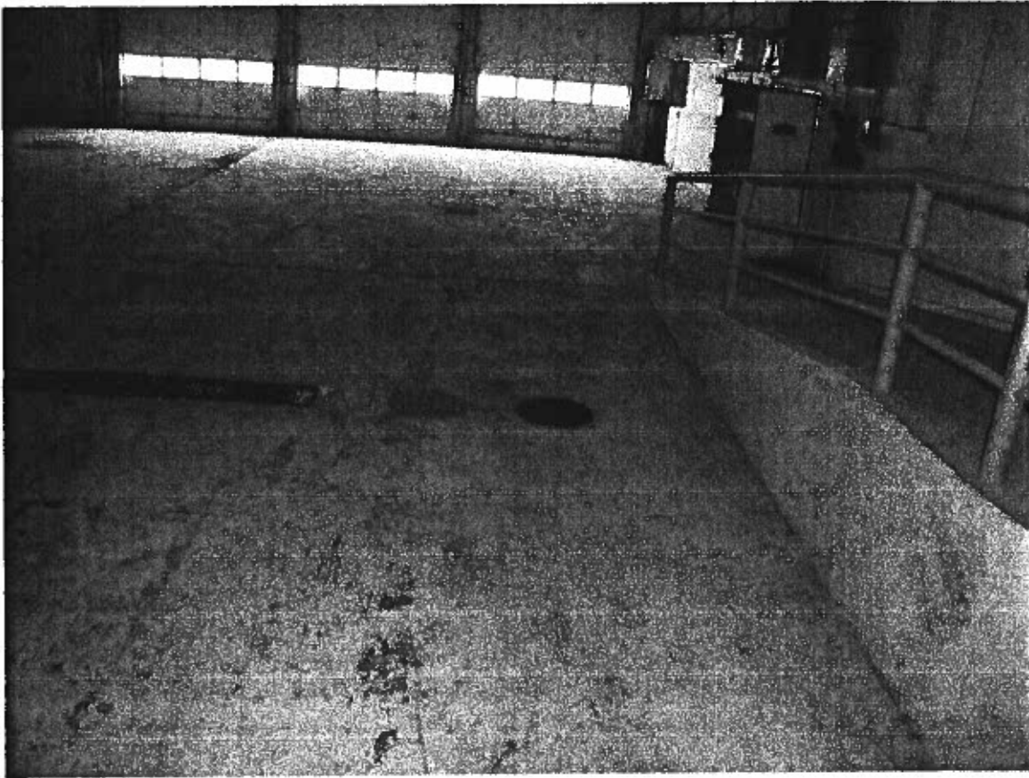
PHOTO 4: Strip floor drain and oil/water separator/sediment trap in North bay of warehouse/shop building.
