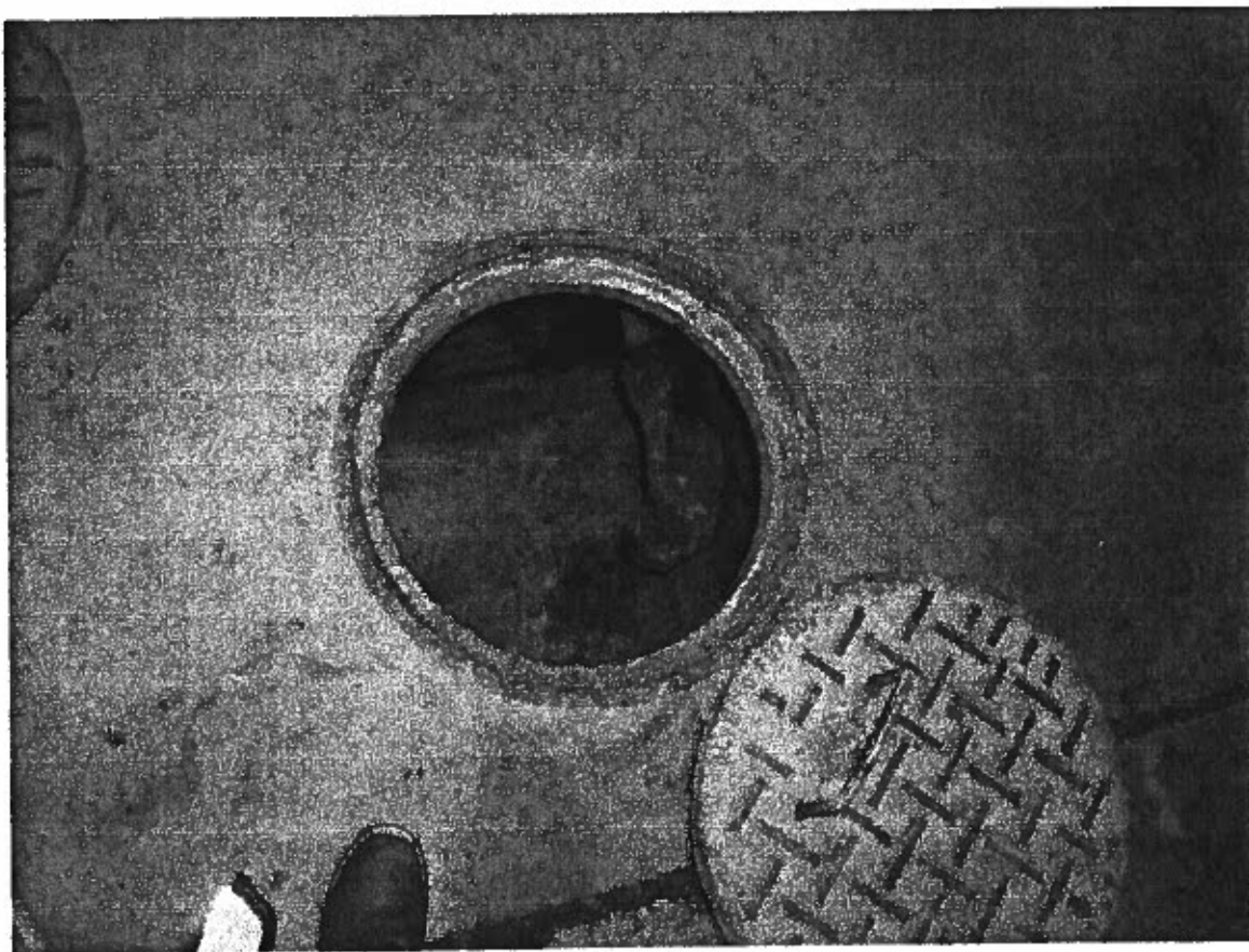
PHOTO 3: View into oil/water separator/sediment trap in South bay of warehouse/shop building.
