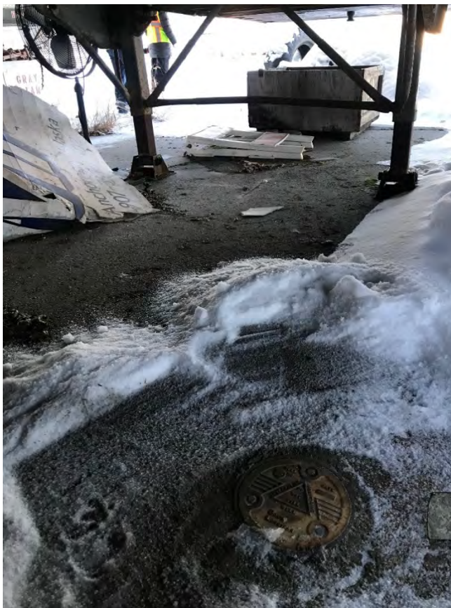
Photo No. 2 – 15 December 2020
