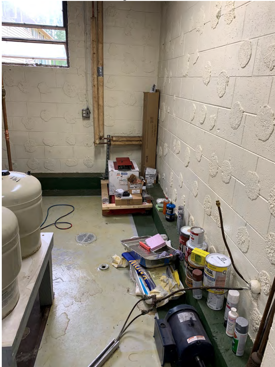
Photo 1. Interior of boiler room facing south
