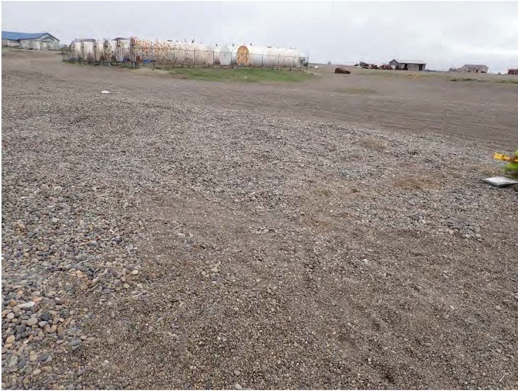
Photograph 5: GPS location of well 16GAMMW05 is within this area of gravel that differs from surrounding gravels. It is evident that there was once a larger gravel pile in this area. Heavy equipment used to move this gravel may have damaged or removed the well.
