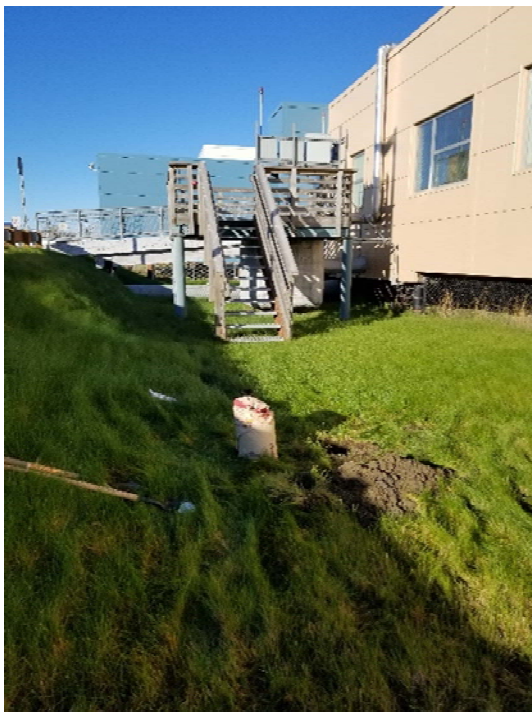
MW-8 Location and Bentonite
