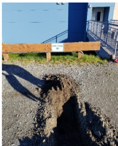
Excavation at MW-3 to Expose Top of Casing
