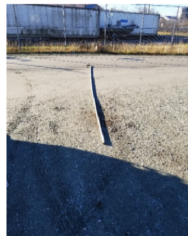
Removed MW-3 Casing
