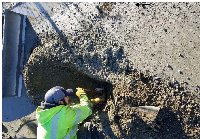
Connecting Bolt to MW-1 Well Casing for Removal
