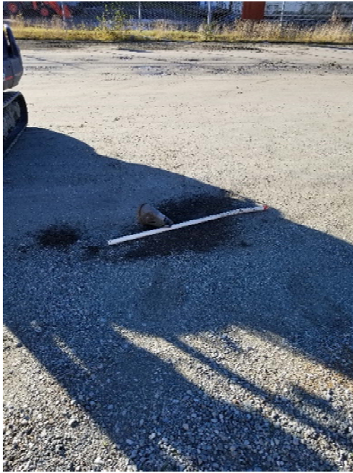
Broken MW-4 Casing
