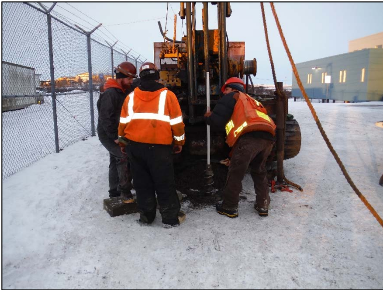
Installation of MW-1
