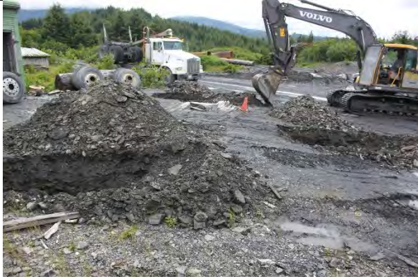
Photo showing Test Holes dug outside the Equipment Shed.
