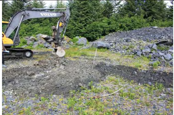
Photo showing the drive-point monitoring well installed at TH27.
