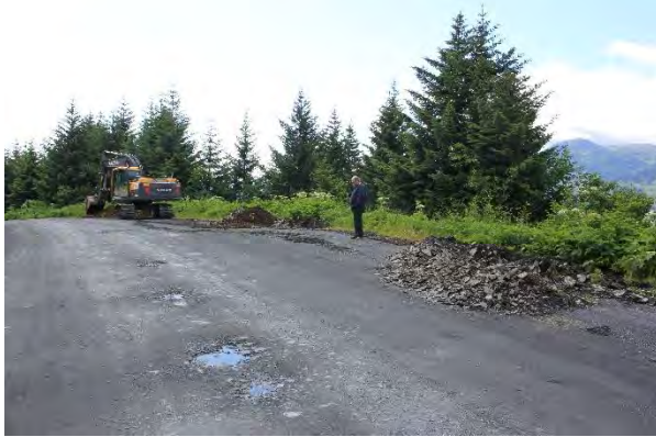
Photo showing the Test Holes at 1.0 Mile Road Saw Gas site.
