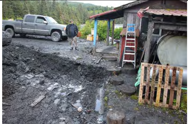
Photo showing TH23 which was dug in front of above-ground storage tanks.
