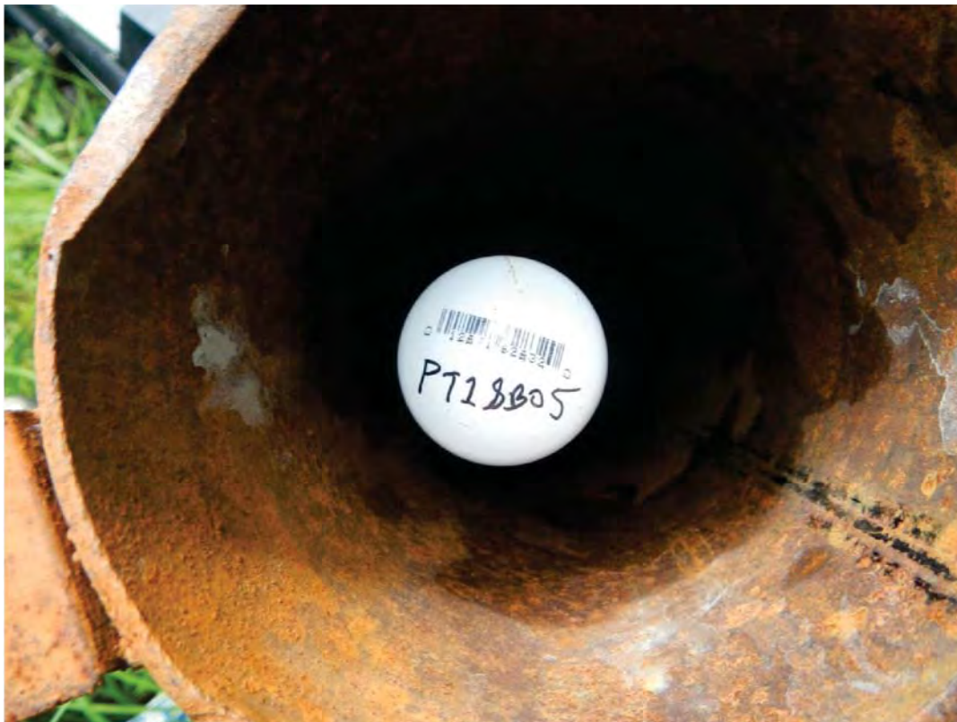
Photo 8: Site OT001, Subarea PT1, well PT1SB05; view of replaced well cap.
