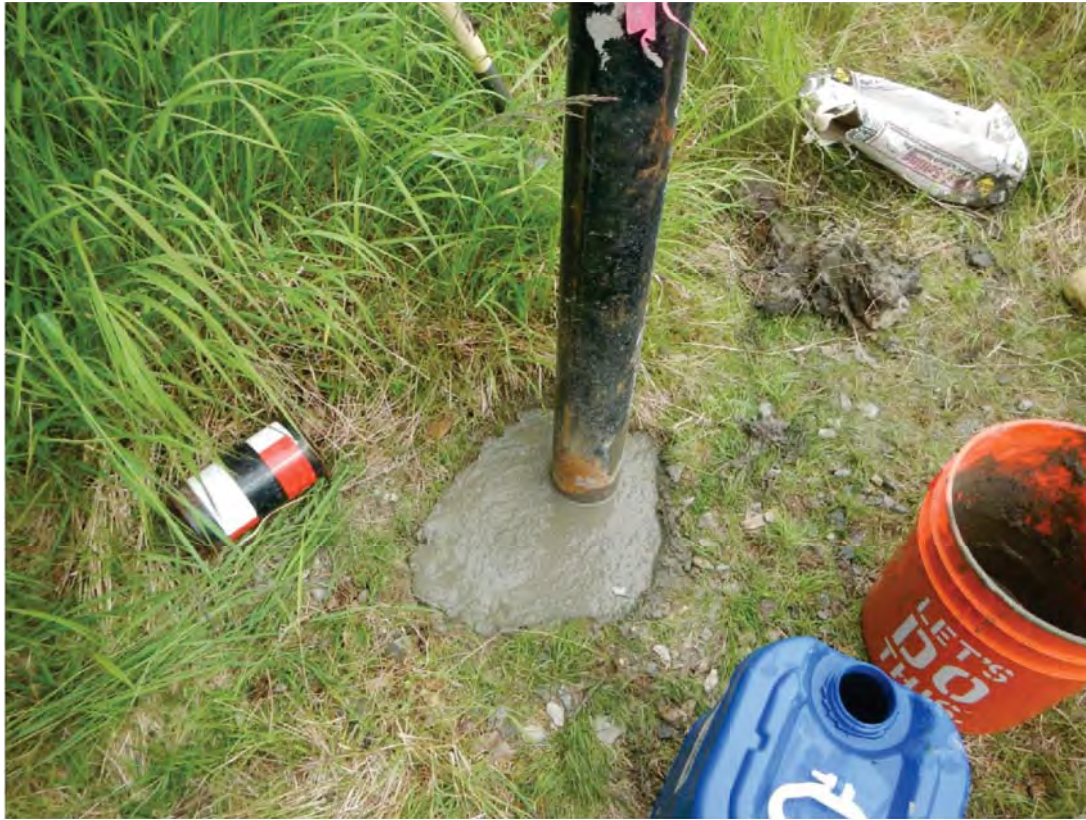
Photo 7: Site OT001, Subarea PT1, well PT1SB04; view of 2014 repaired condition.
