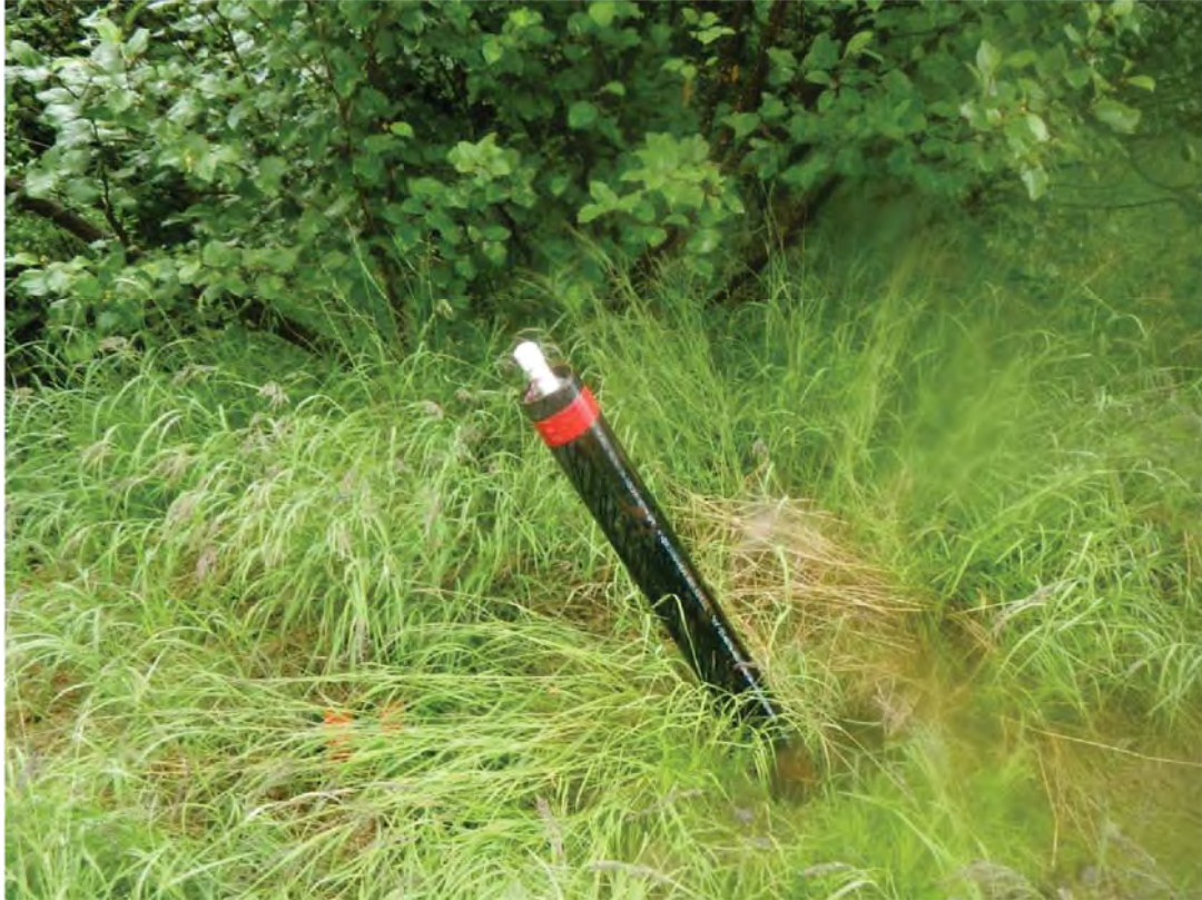
Photo 9: Site OT001, Subarea PT1, well PT1SB15; view of pre-repair condition.
