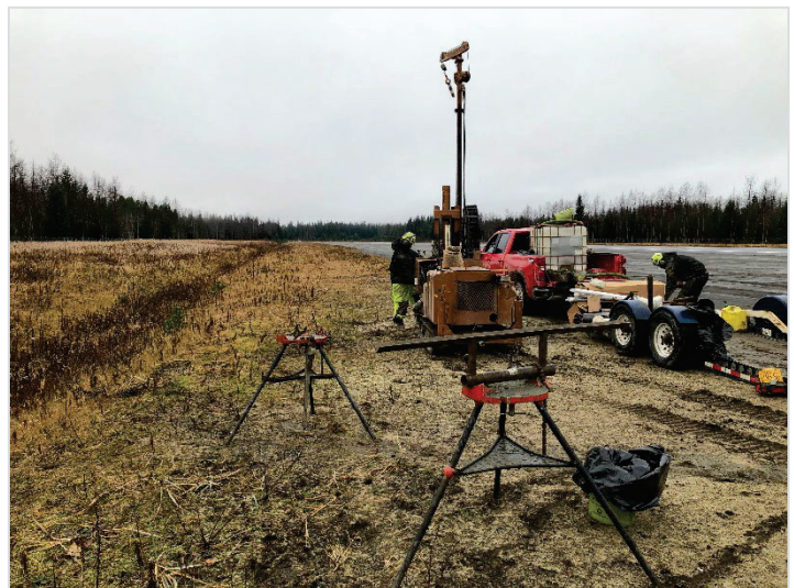
Exhibit 2-1: Drilling at Runway near the ARFF building
