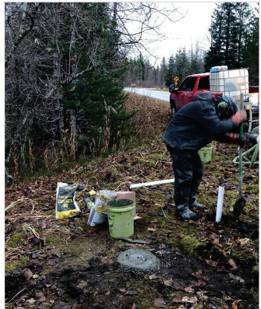
Exhibit 2-2: Well installation at MW-22
