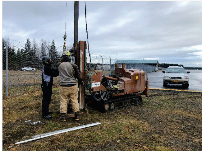
Exhibit 4-1: Drilling near the Alaska Airlines terminal
