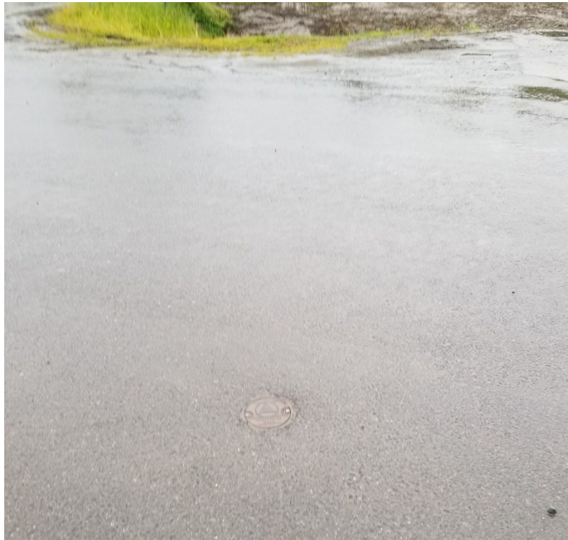
Photo 2: Monitoring well MW4a with new surface monument. September 10, 2021, facing south.
