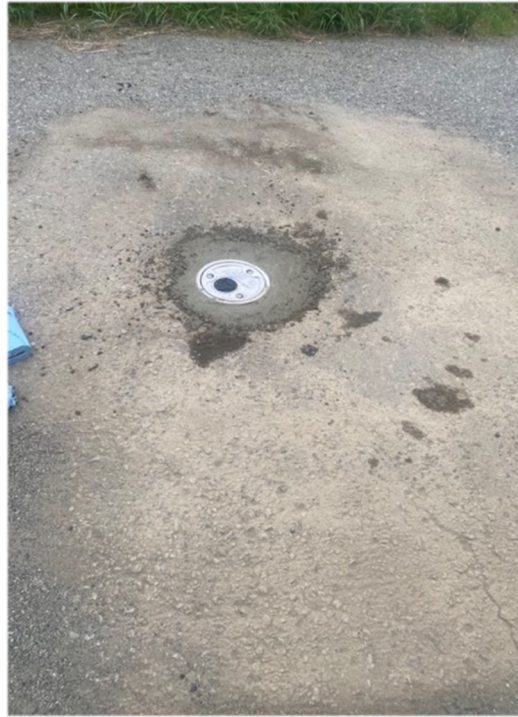
Photo 5. MW-6 after completion of repairs.
