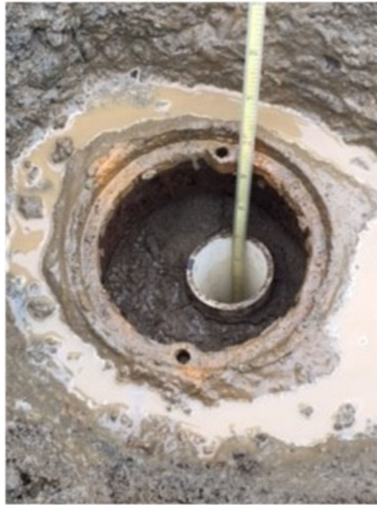
Photo 3. Monitoring Well (MW)-4. MW-1, MW-3, MW-5, and MW-6 are of similar construction.
