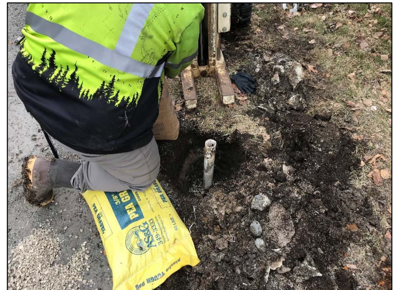
MW-4, view is close up
