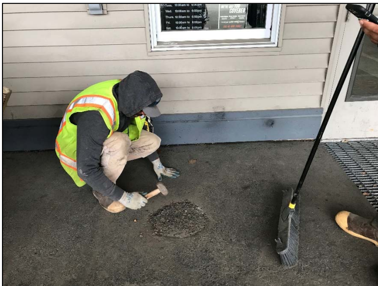
MW-2, view is south
