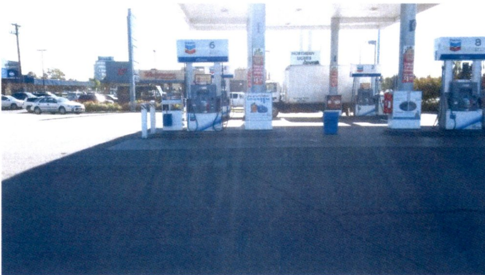
Photo 5 – View of site looking south
