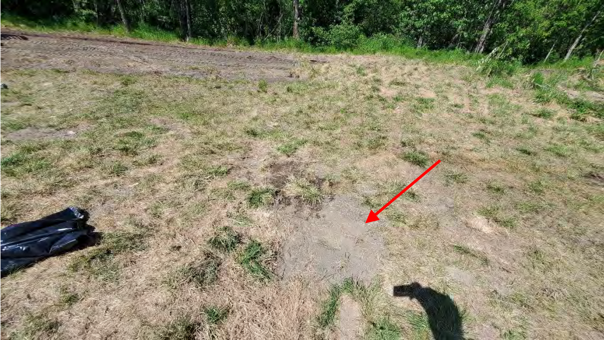
Photograph #3 – 6 June 2022. Decommissioned monitoring well MW1A (marked with a red arrow) after backfilling the soil above the pea gravel. View facing northwest.
