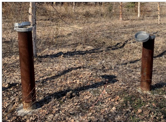
Exhibit 6-1: Collocated monitoring wells MW-17 and MW-27; from left to right.
