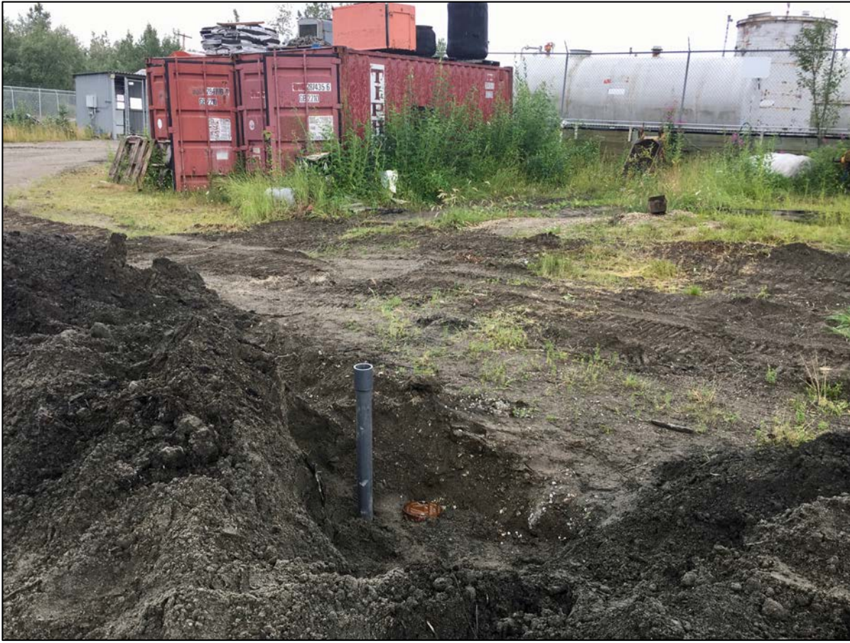
Photo: 7 Date: 8/2/2018 Direction: North Subject: Completed flush mount well.
