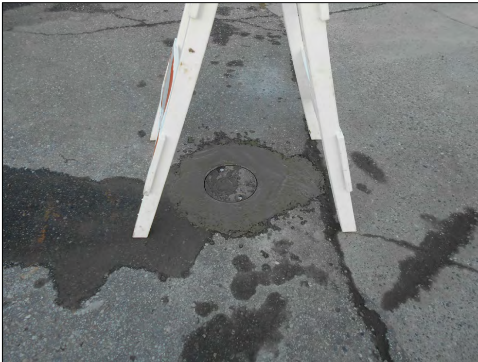
Photograph 16: New Well Cover at VMP-2, Former Park-n-Sell Lot
