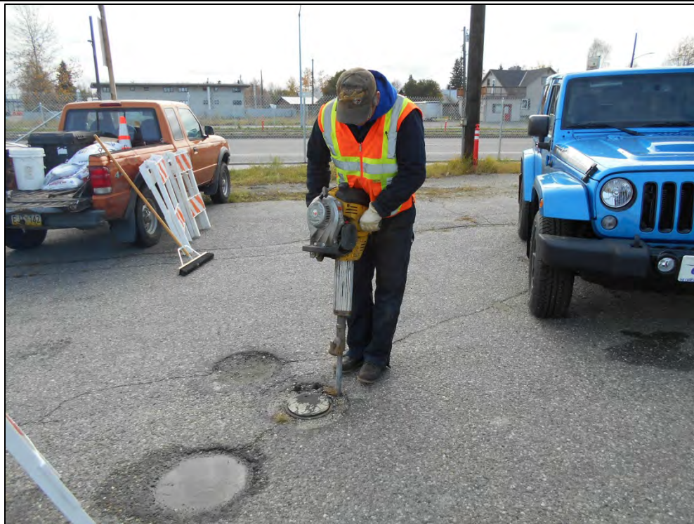
Photograph 14: Removing Former Concrete Around MW-29S, Former Park-n-Sell Lot
