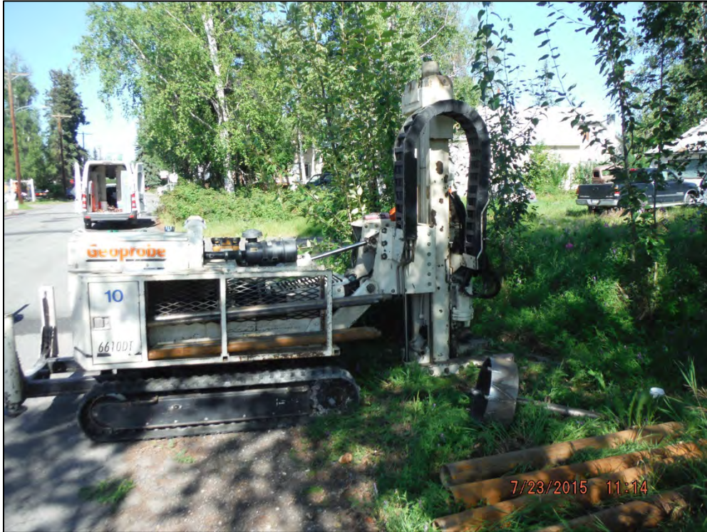
Photograph 5: Installing VMP-7 on 8 th Ave. Right-of-Way
