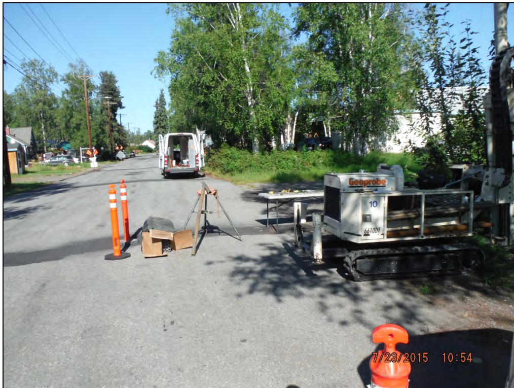
Photograph 4: Installing VMP-7 on 8 th Ave. Right-of-Way
