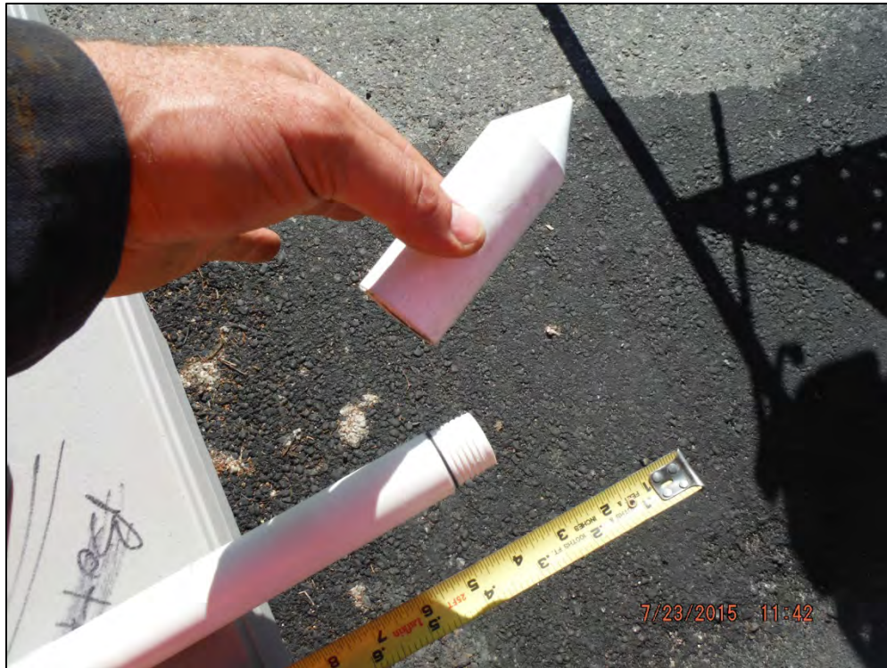
Photograph 1: Bottom Cap on 1-inch Sch 80 PVC VMPs
