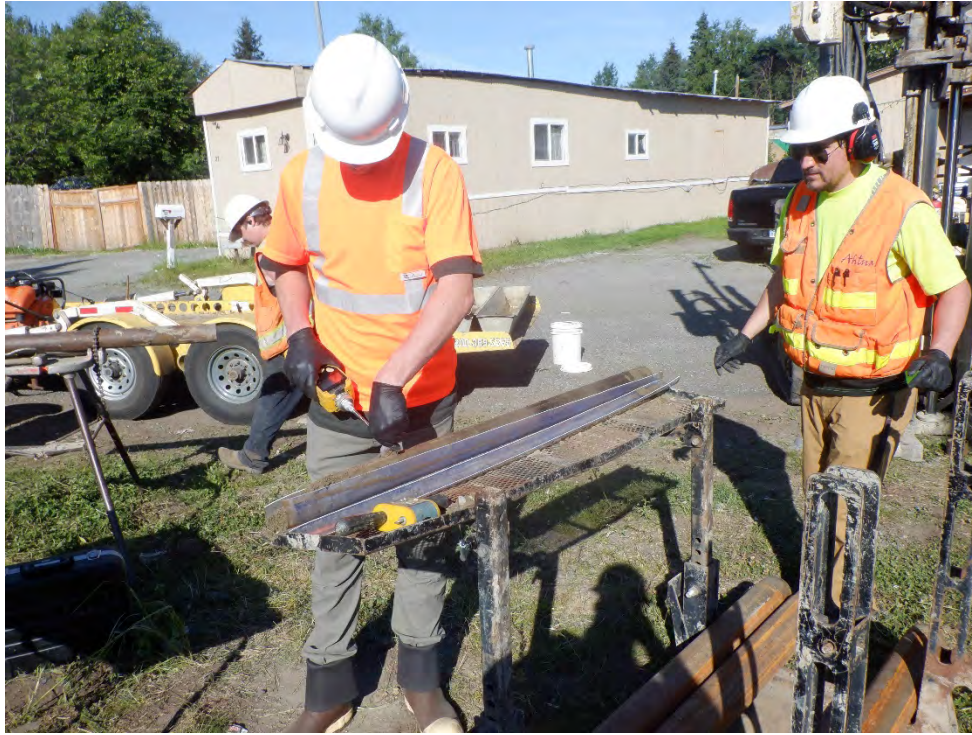
Photograph 11: PID screening soils for monitoring well installation. View west.
