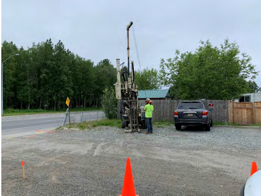
Photograph 9: Drilling at soil boring location SB-7. View southwest.
