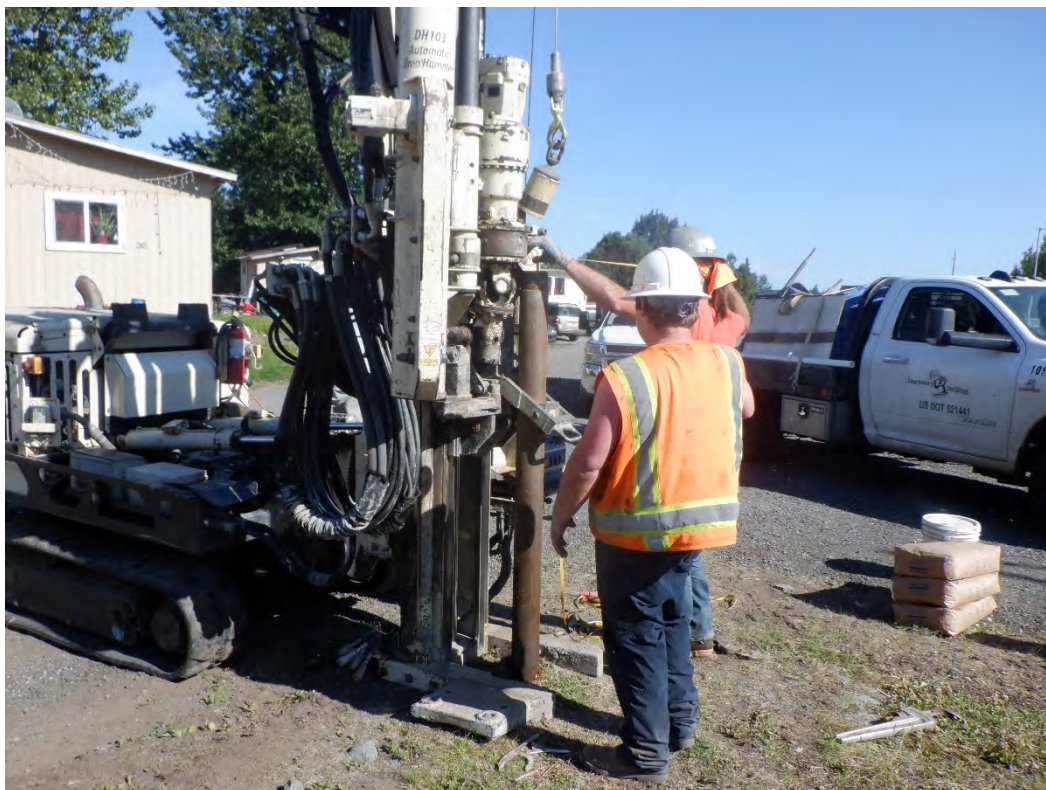
Photograph 10: Drilling at the location for MW-128. View north.
