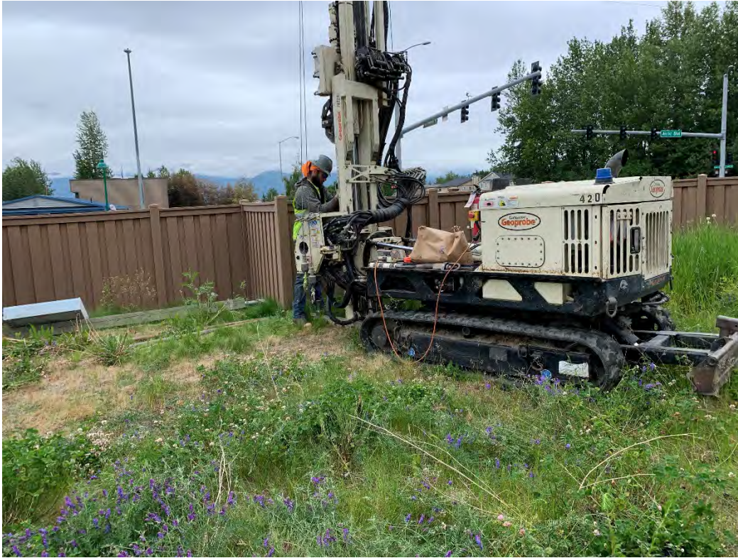
Photograph 7: Drilling at location SB-6. View east.
