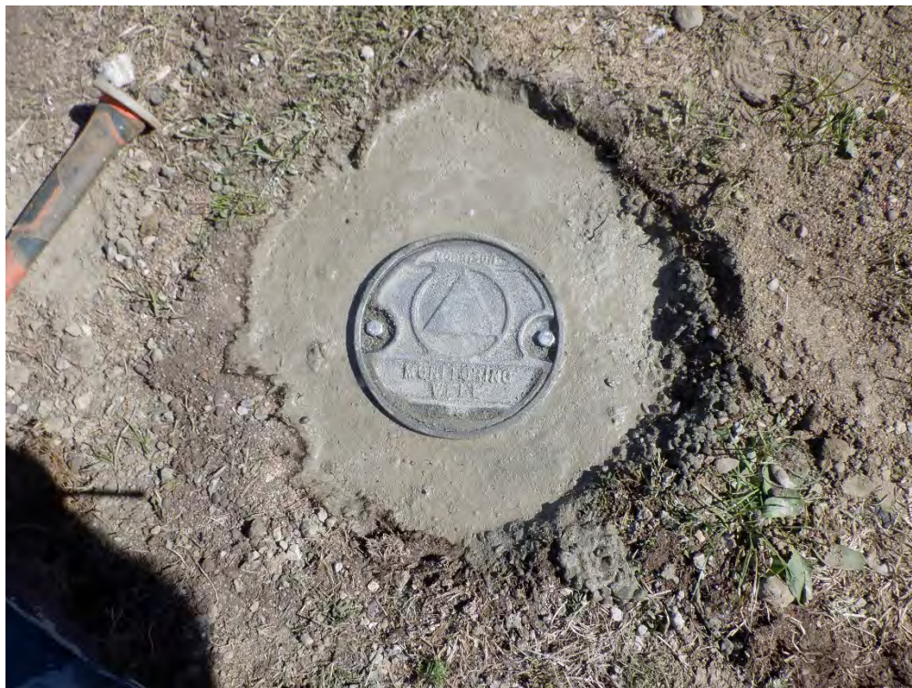
Photograph 14: Completed monitoring well MW-128. View close-up.
