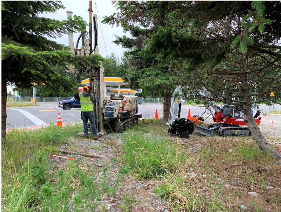
Photograph 3: Drilling at the new location of SB-10. View south.
