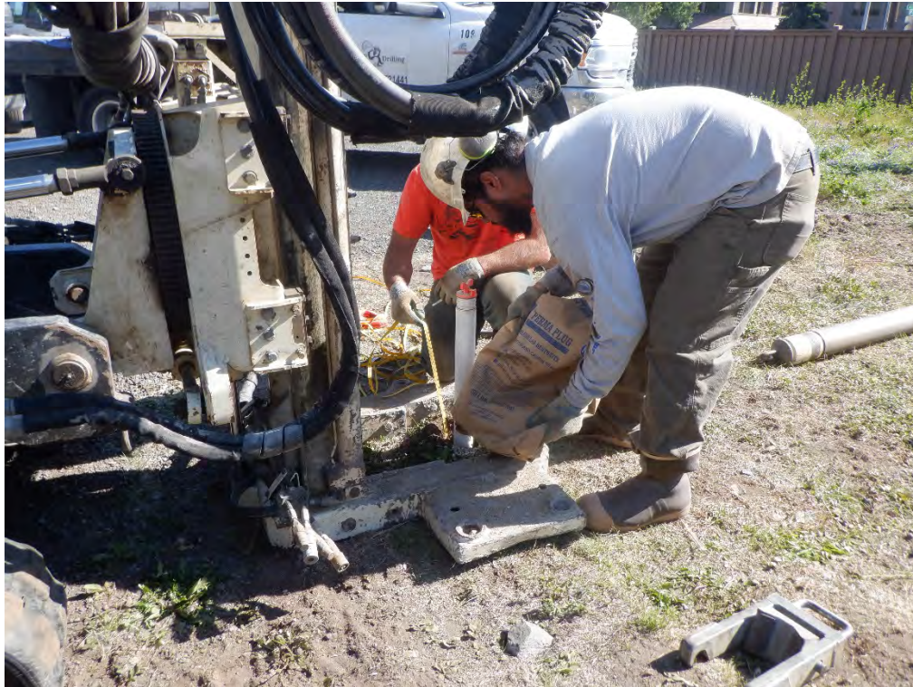
Photograph 13: Installing monitoring well MW-128. View close-up.
