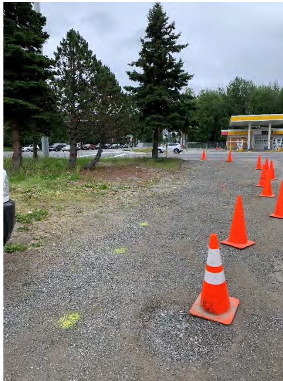
Photograph 4: Soil borings SB-4 and SB-8 at staked locations in road. Locations were moved slightly to the west to avoid gas utility marked in yellow paint. View south.
