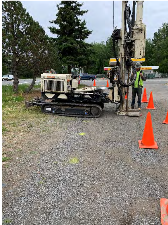
Photograph 5: Drilling at soil boring location SB-04. View south.
