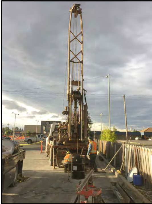
PHOTO 3 - DISCOVERY INSTALLING WELL MW-3
