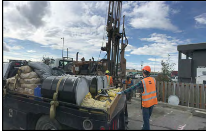
PHOTO 5 - DISCOVERY INSTALLING MW-1
