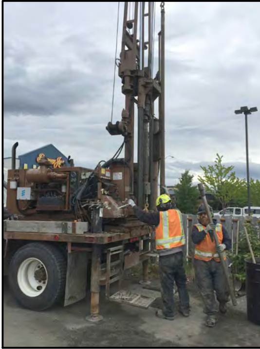
PHOTO 1 - DISCOVERY DIRECT-PUSH DRILLING OF WELL MW-4 FOR LITHOLOGY
