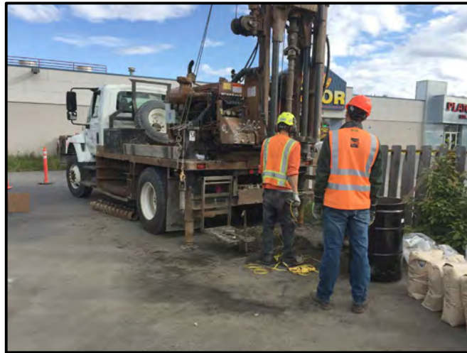
PHOTO 6 - DISCOVERY INSTALLING WELL MW-4
