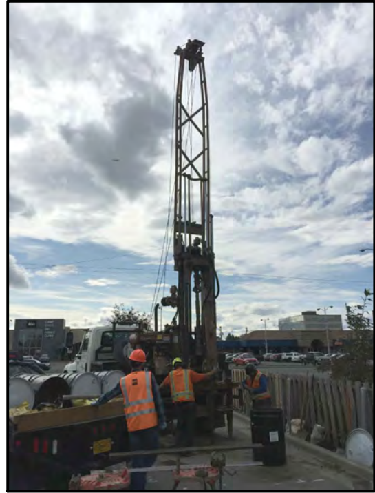
PHOTO 2 - DISCOVERY INSTALLING WELL MW-1
