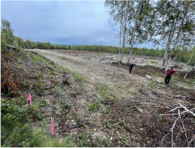
Photo 13: 20220824 looking NE complete
