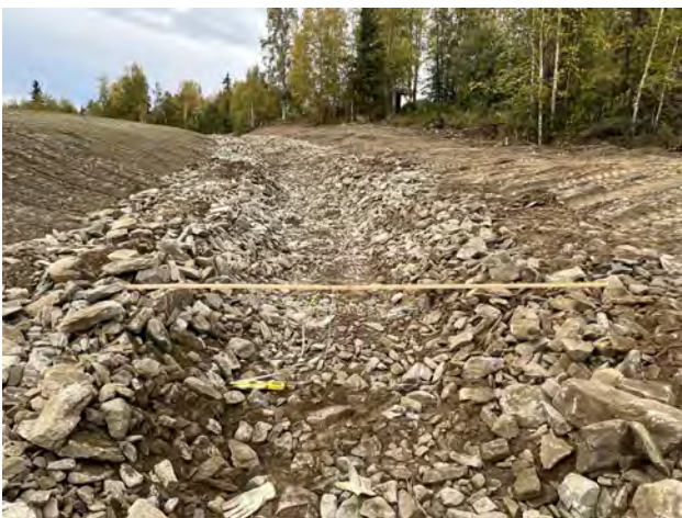
Photo 17: 20220916 upper portion of channel
