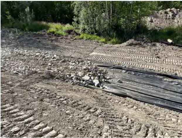
Photo 9: 20220723 Placing Riprap looking west
