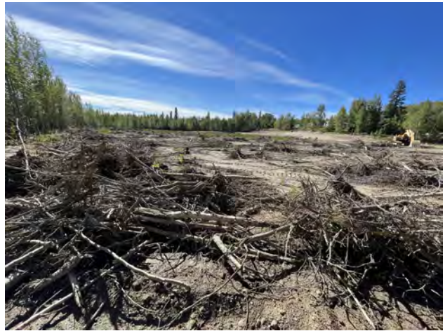
Photo 10: 20220811 Final Surface looking south
