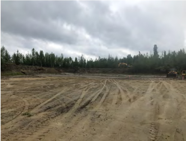
Photo 1: 20210728 Initial Lifts looking south
