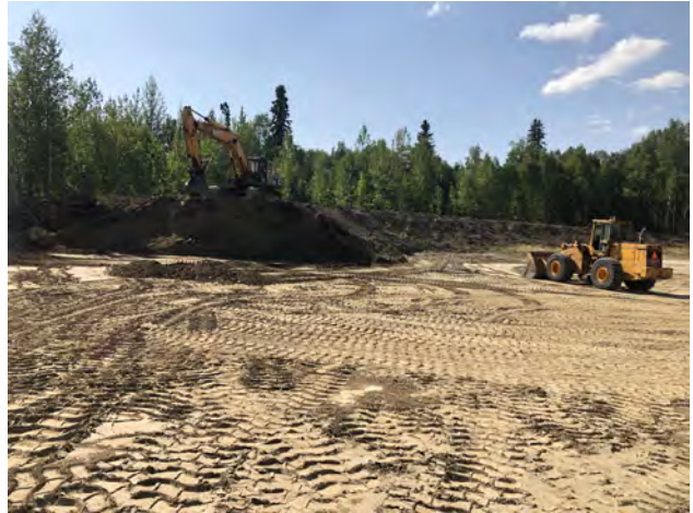
Photo 2: 20210804 Dismantling southern berm
