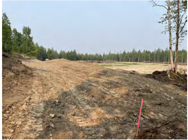
Photo 8: 20220630 Beginning of Diversion Ditch looking North
