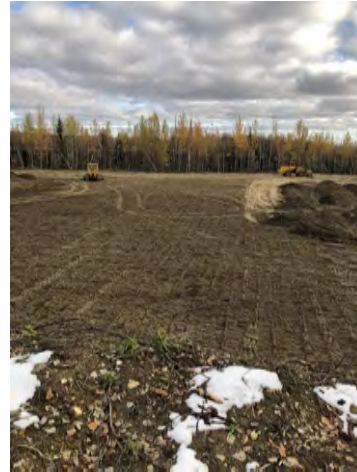
Photo 4: 20210927 final surface looking east
