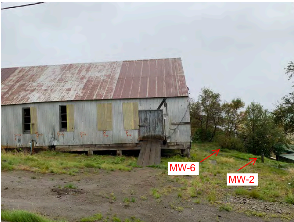
Photo 4: SE Side of Fisherman Gear Building, MW-2, and MW-6. September 6, 2019.
