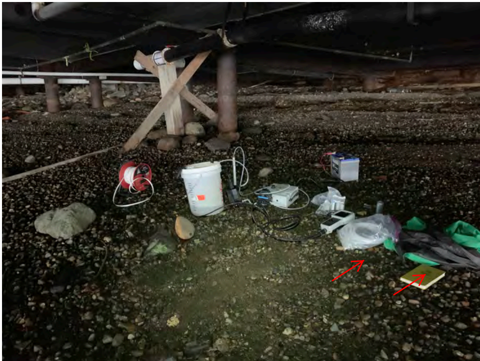
Photo 6: Sampling at Temporary Well Point MW-5R. September 7, 2019.
