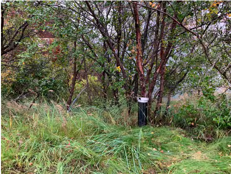
Photo 8: Monitoring Well MW-7. September 9, 2019.
