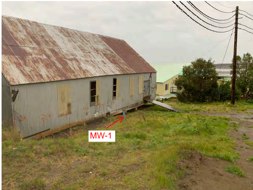
Photo 3: SW Side Fisherman Gear Building, Monitoring Well MW-1. September 6, 2019.
