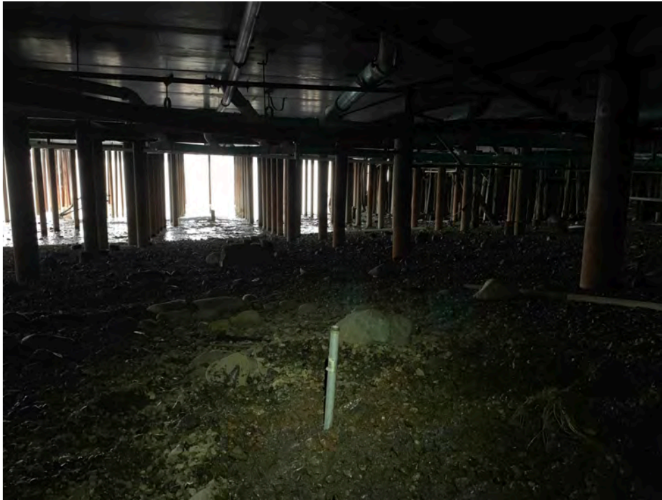
Photo 5: Temporary Well Point MW-5R Beneath Cold Storage Building. September 7, 2019.
