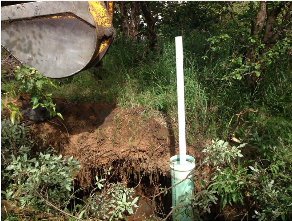
Photo 7: Installing monitoring well MW-2
