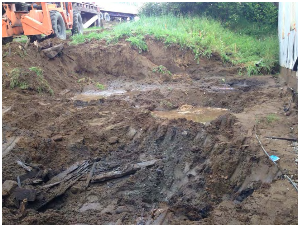
Photo 2: Poned areas mid-excavation
