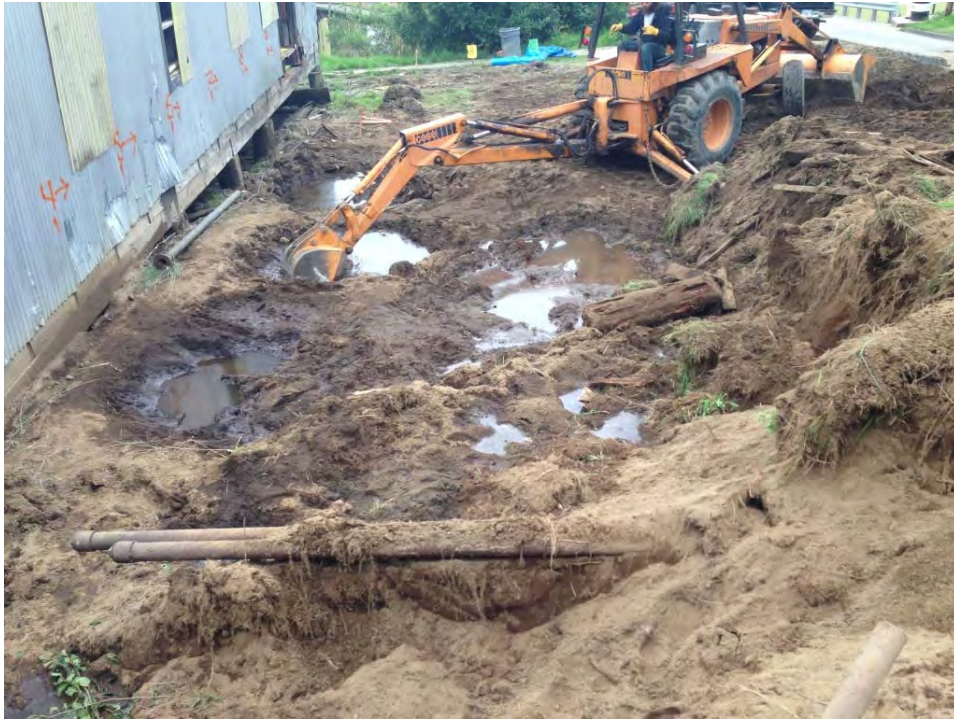
Photo 5: Excavating monitoring well MW-1, photo facing south.
