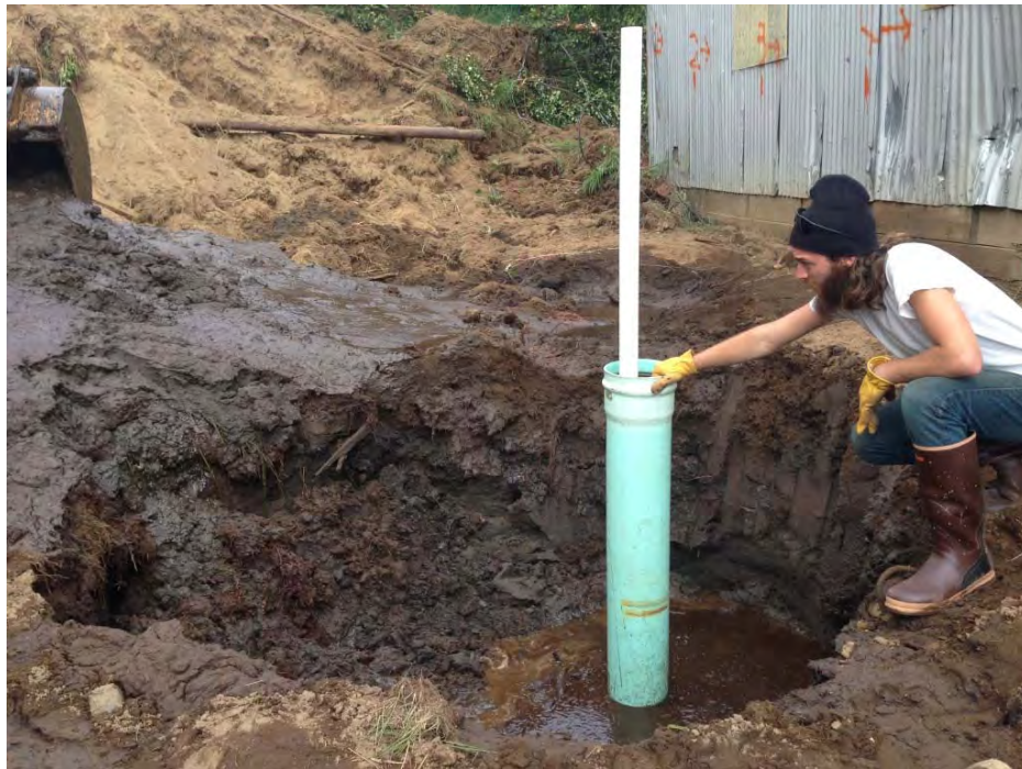
Photo 6: Installing monitoring well MW-1
