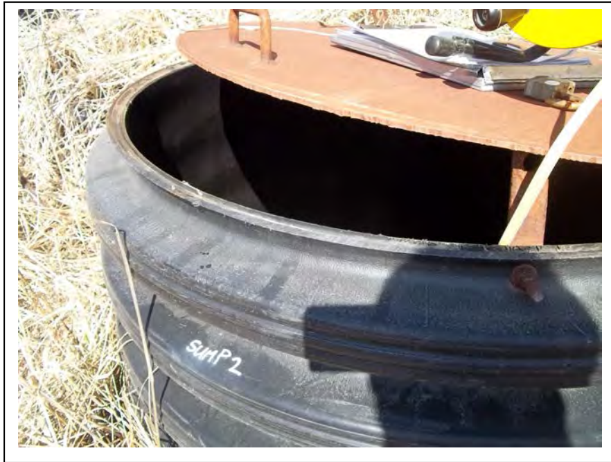
Photo 20: Sump 2 was in good condition. (May 12, 2014)
