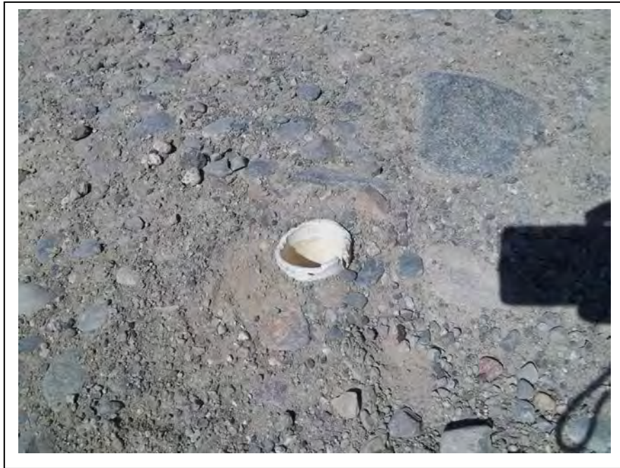
Photo 6: Monitoring Well MW-2 was missing its protective monument and well cap, and was filled with about 3 feet of soil. (May 12, 2014)
