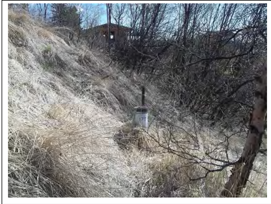
Photo 18: Monitoring Point MP5 was in good condition. (May 12, 2014)
