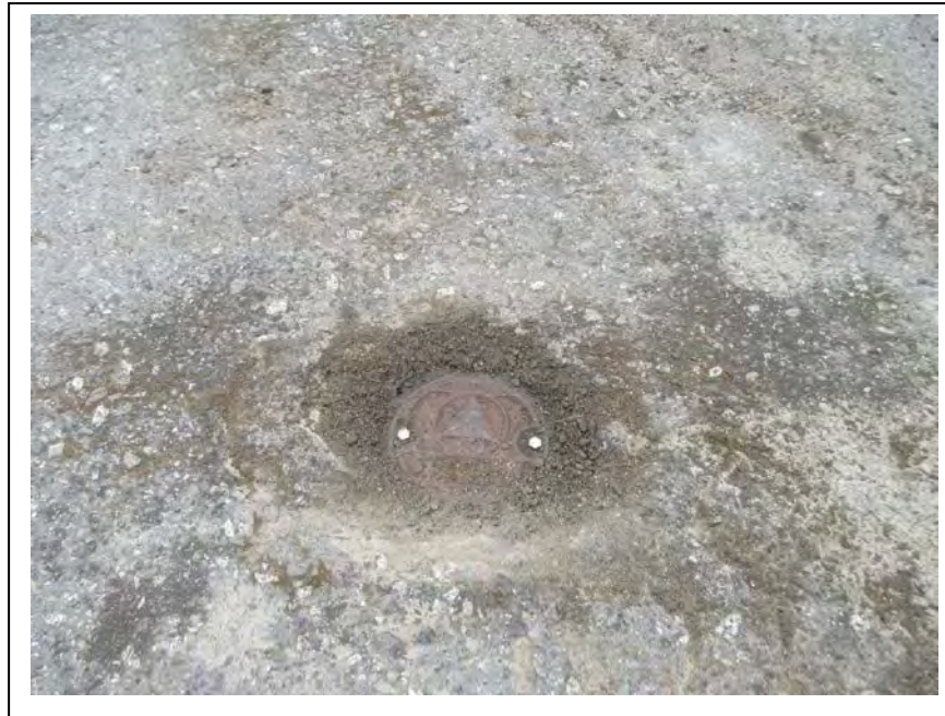
Photo 26: Monitoring Well MW-6 after repairs on June 11, 2014. (June 11, 2014)
