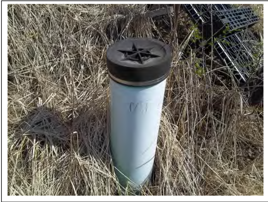
Photo 17: Monitoring Point MP4 was in good condition. (May 12, 2014)
