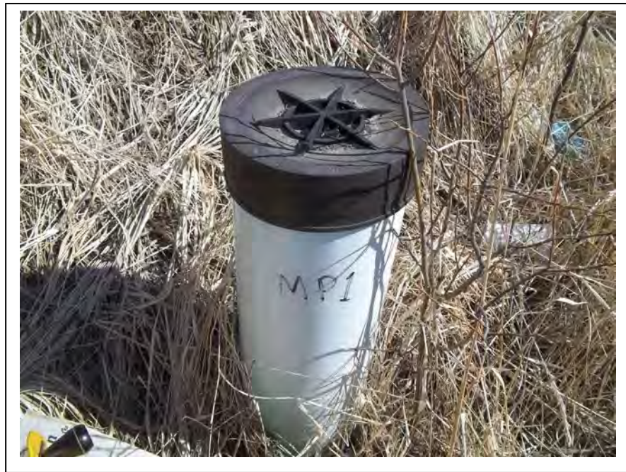
Photo 14: Monitoring Point MP1 was in good condition. (May 12, 2014)
