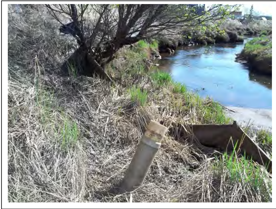
Photo 21: Recovery Well R6 was dry and frost-jacked. (May 12, 2014)
