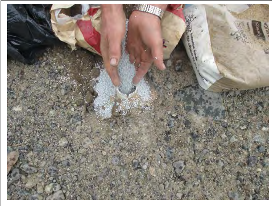
Photo 25: Monitoring Well MW-2 was decommissioned on June 11, 2014. (June 11, 2014)
