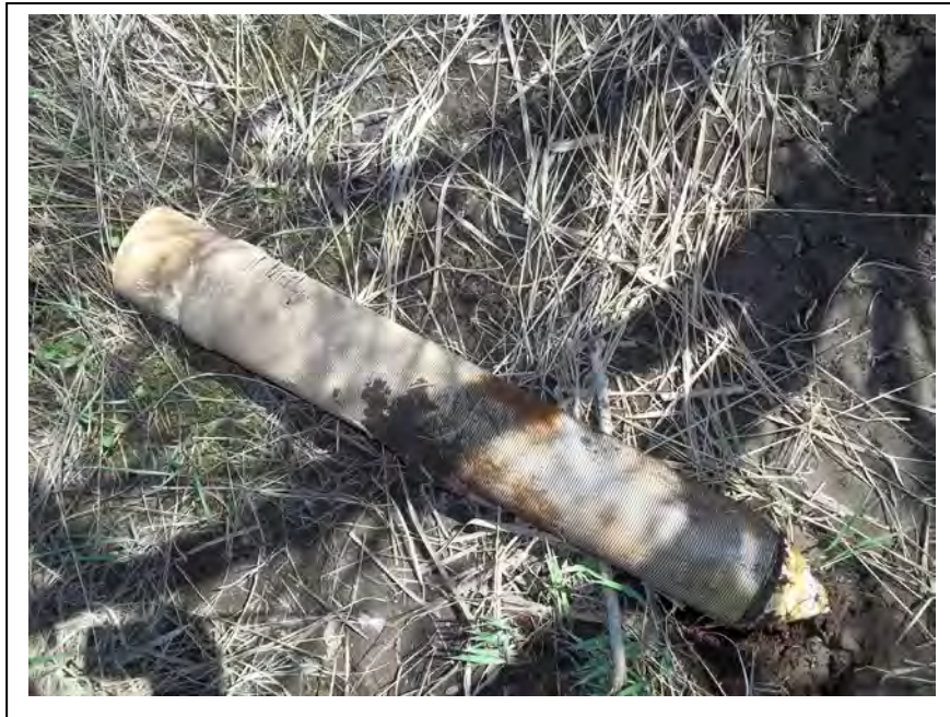
Photo 22: Recovery Well R7 was dry. The well was removed from the ground to help identify it and was decommissioned the following day. (May 12, 2014)
