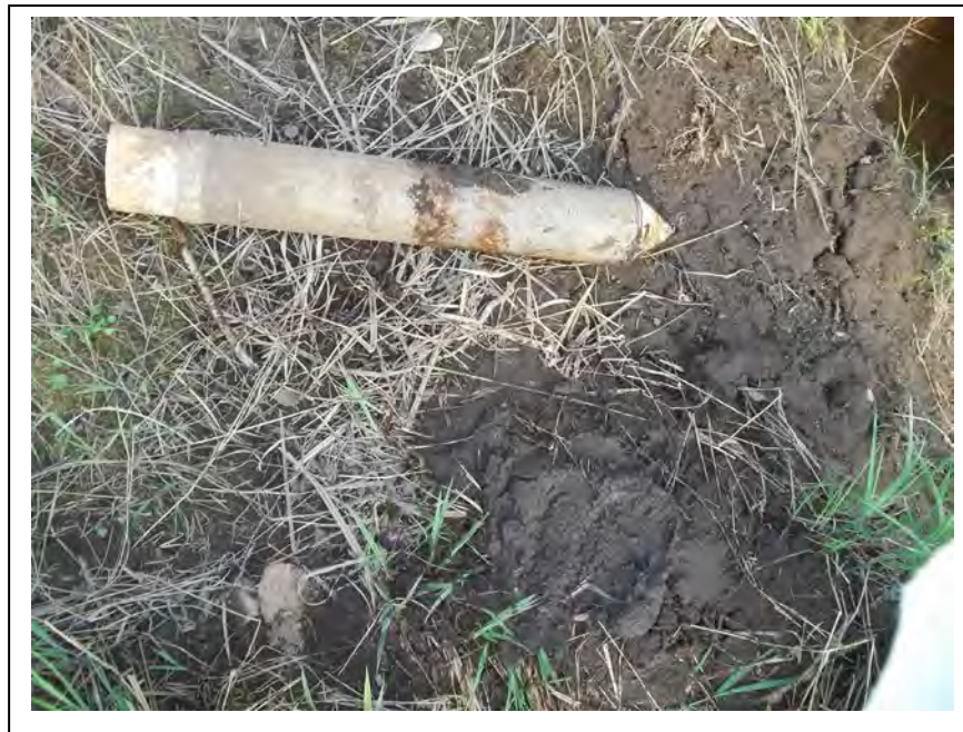
Photo 24: Recovery Well R7 was decommissioned on May 13, 2014 by removing the well from the ground and filling the hole with nearby soil. (May 13, 2014)
