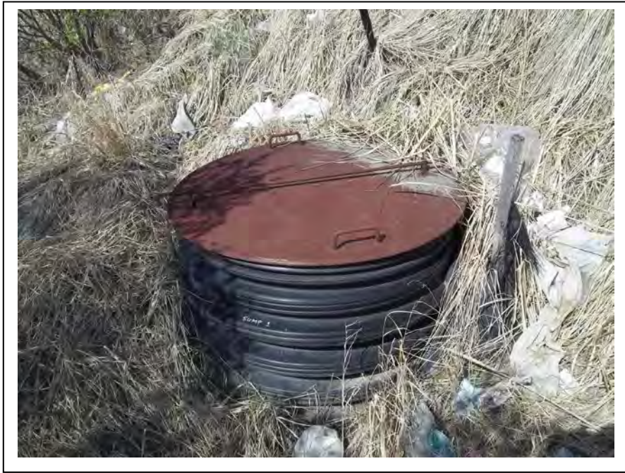
Photo 19: Sump 1 was in good condition. (May 12, 2014)
