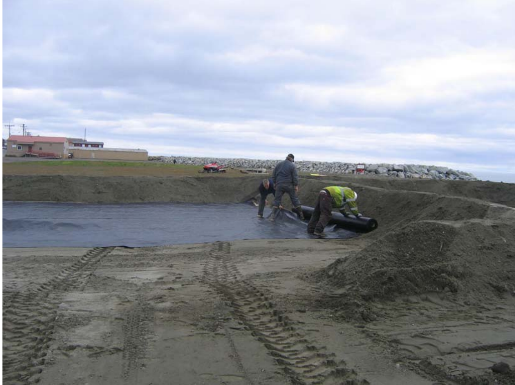
Figure 2: Laying foundation plastic for the soil stockpile.
