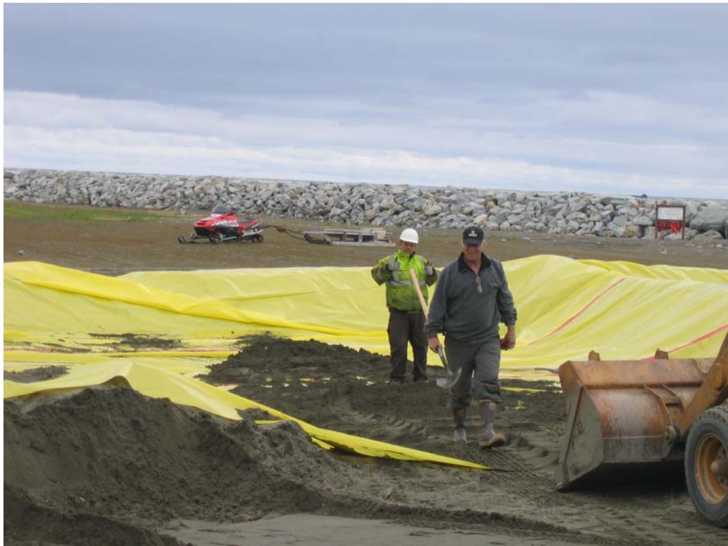
Figure 3: A tarp over the black plastic for the soil stockpile.
