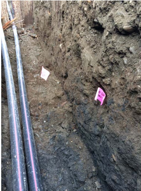
Sampling Points Flagged in Utility Trench
