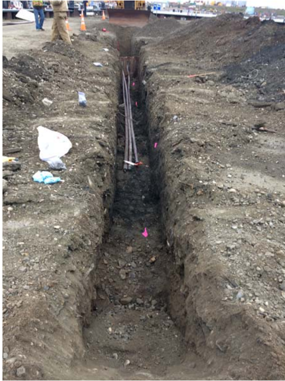
Sampling Points Flagged in Utility Trench
