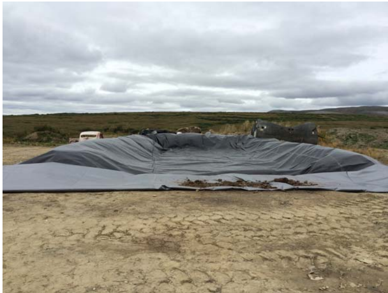
Contaminated soil stockpile area
