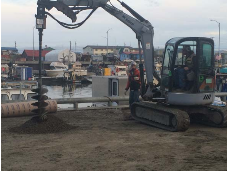
Auguring Light Poles
