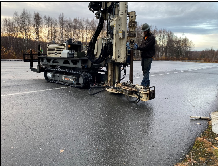
Installing soil boring RSE-3; looking southeast
