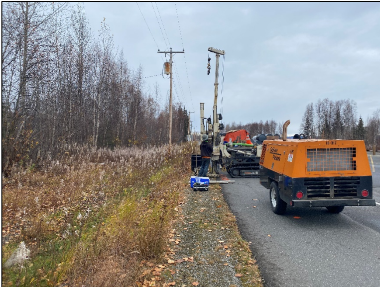
Installing RSE-1; looking north
