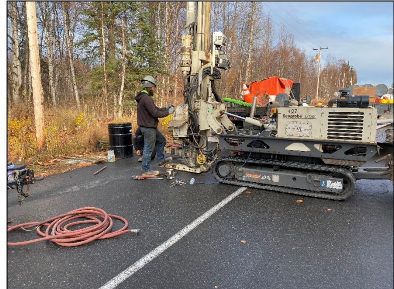
Installing soil boring RSE-2; looking northwest
