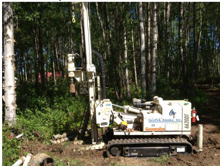
Photo 6. Installing Monitoring Well MW8 (looking north)
