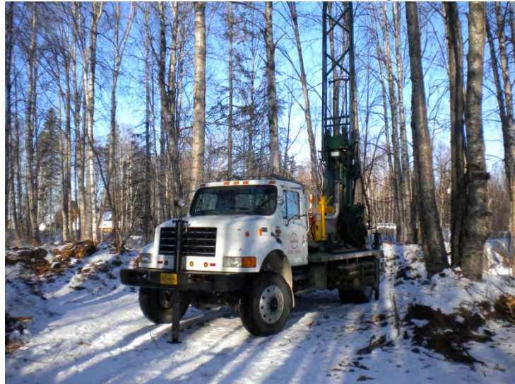
Photo 3. Drilling Soil Boring SB1 (looking northwest)
