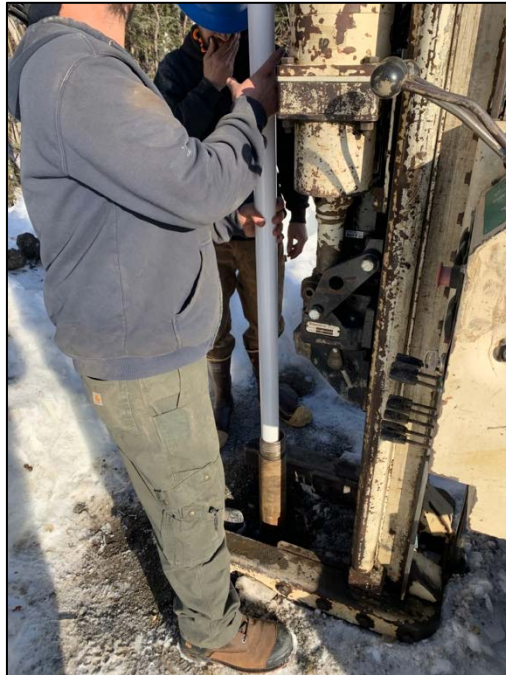
Photo 1. Monitoring well installation. April 19, 2022
