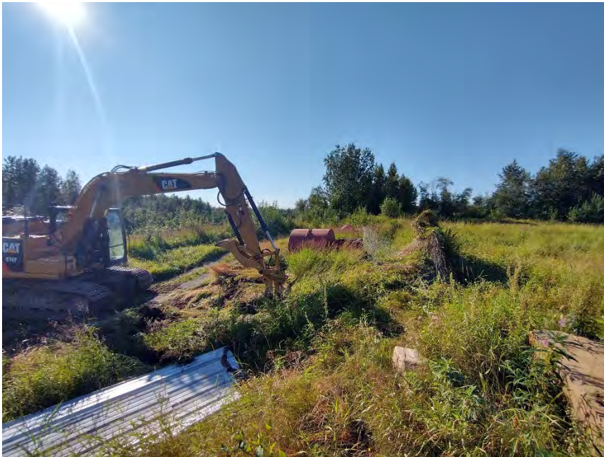
Photo 3: Excavating Test Pit TP2, view south. (August 3, 2021)
