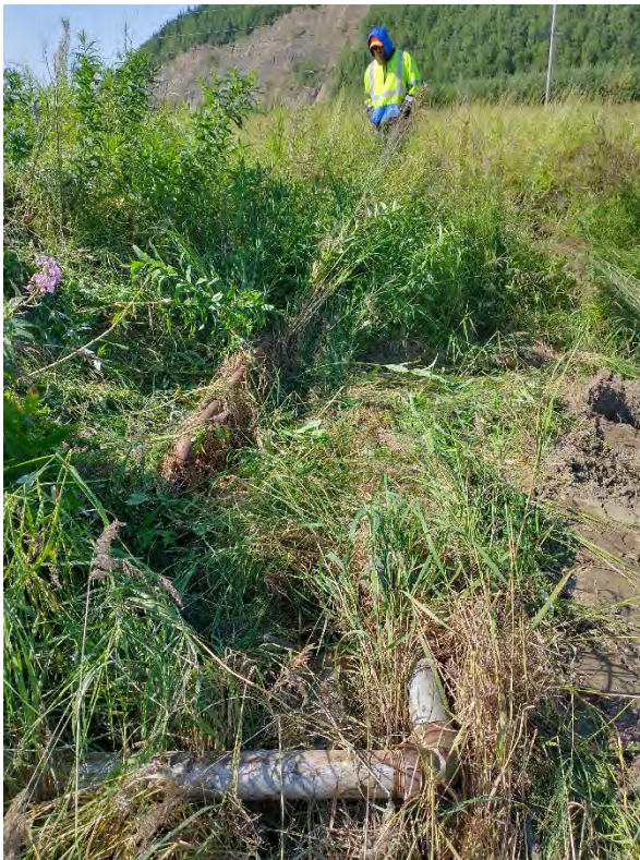
Photo 2: Aboveground piping south of Test Pit 1, view south. (August 4, 2021)
