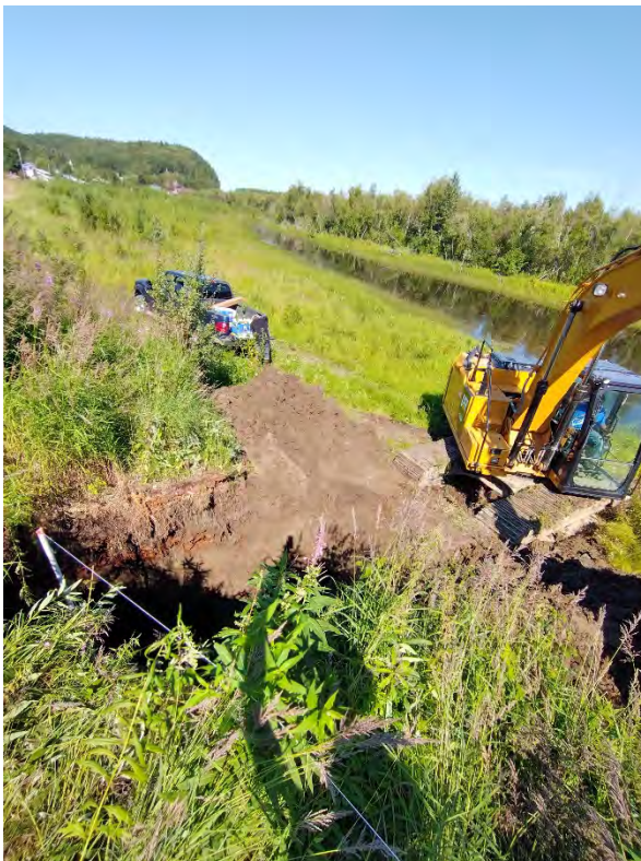
Photo 6: Installing Temporary Monitoring Well TW-TP3, view north. (August 3, 2021)
