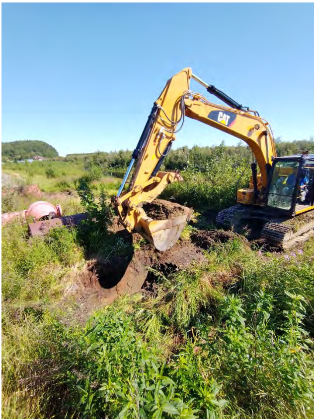
Photo 4: Excavating Test Pit TP1, view northeast. (August 3, 2021)
