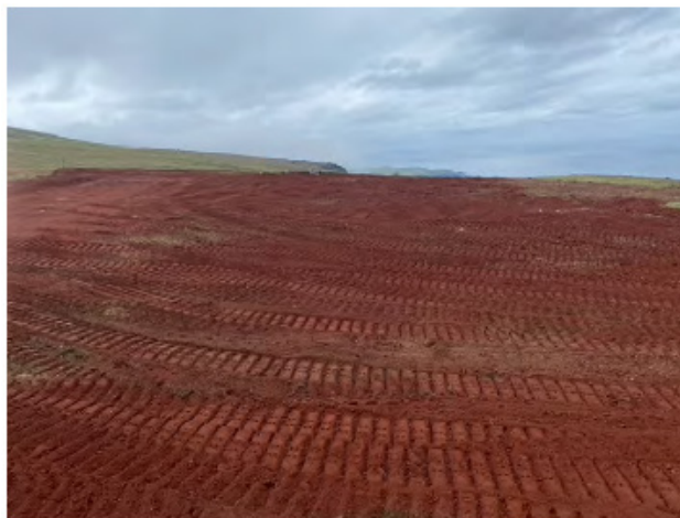
Description: Cap material spread and graded along southern portion of SS02 (Facing west). (6/17/22)
