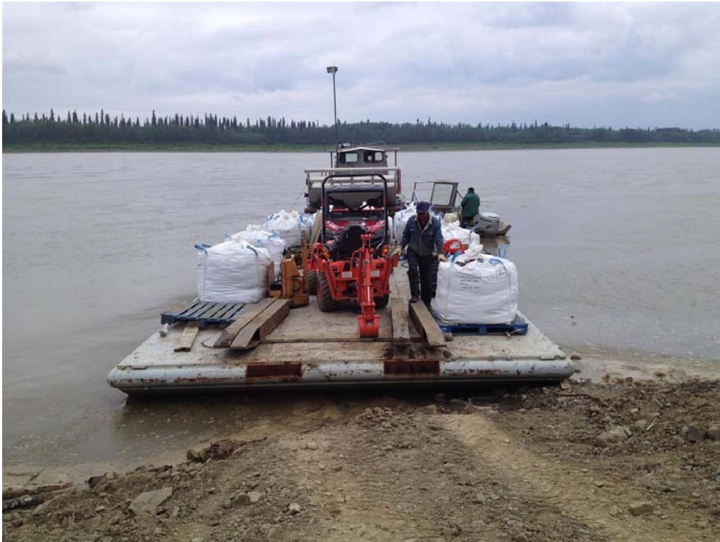
Demobilizing Gear and Supersacks of Excavated Soil
