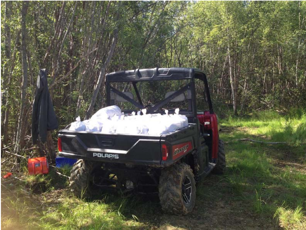
Soils from IA-2 Excavation Prepared for Transport to Barge Landing
