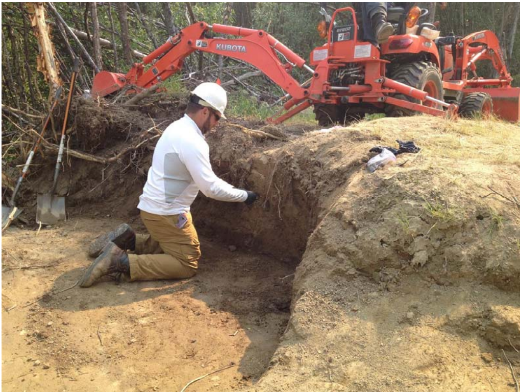
Sampling Soil on Southeast Sidewall at IA-2 Excavation
