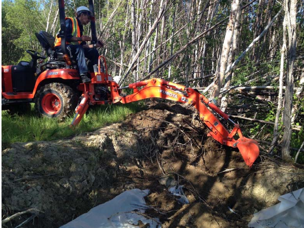
Excavating Soil on Southwest Sidewall at IA-2
