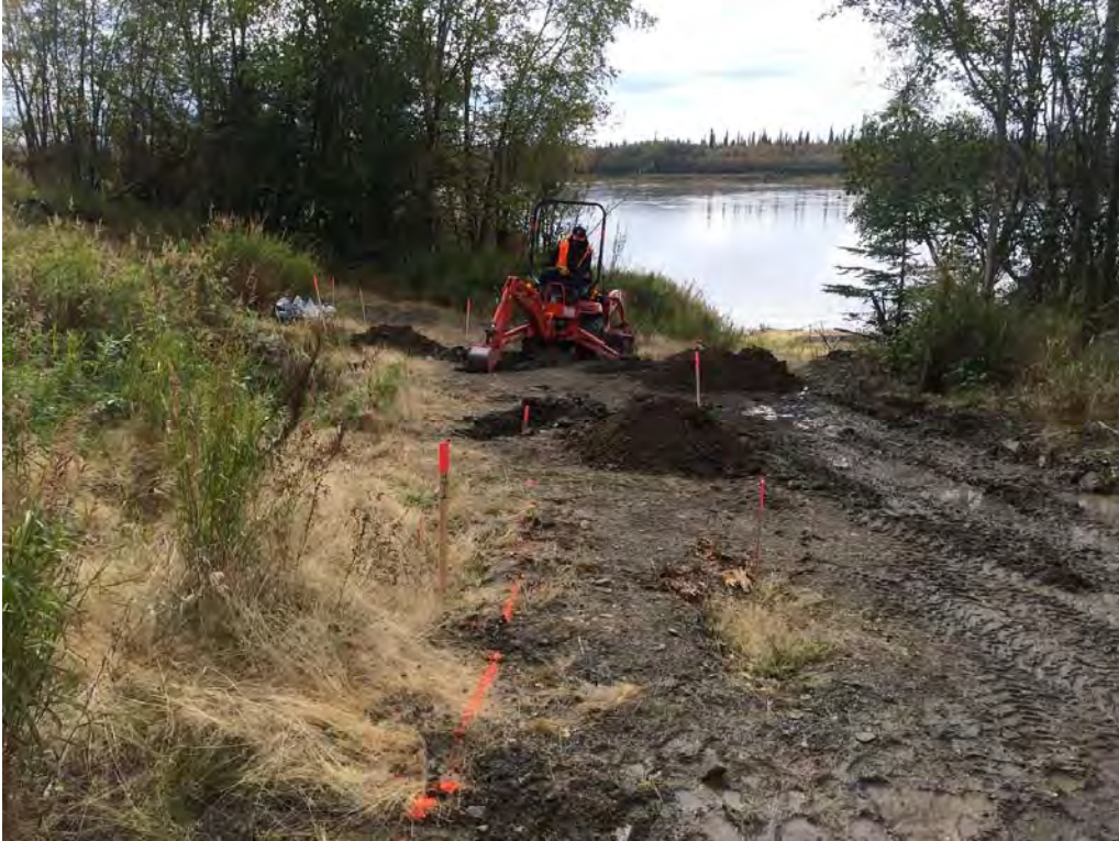
Photo 1 - Excavating at test pit TP-22
