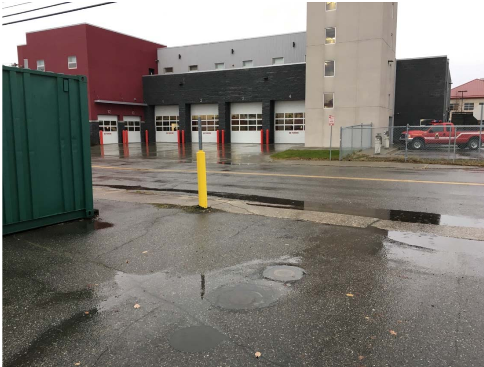
Photo 3: Location of monitoring well MW-34A.
