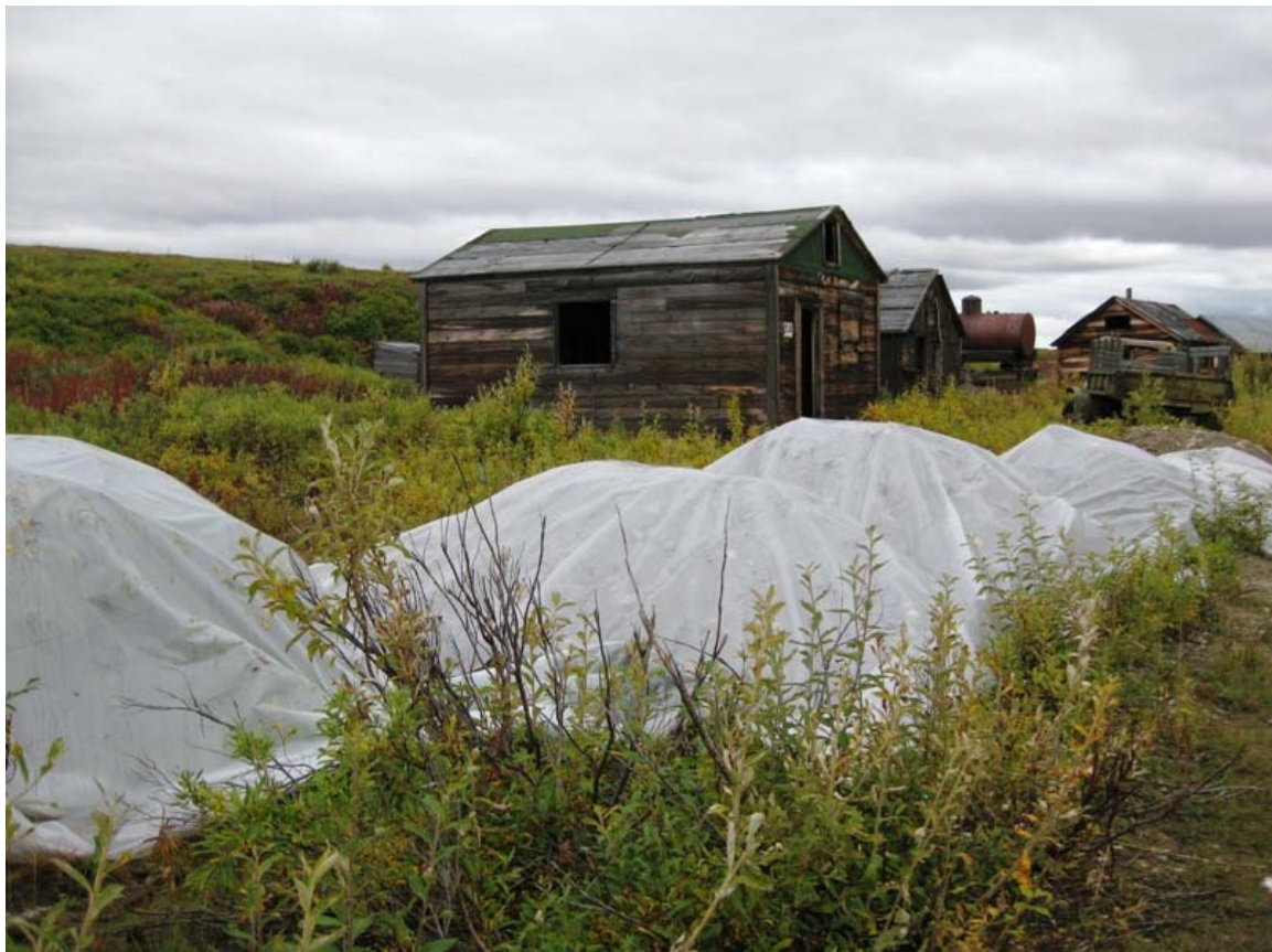
2. Contaminated soil stockpiles located in the upper camp area.
