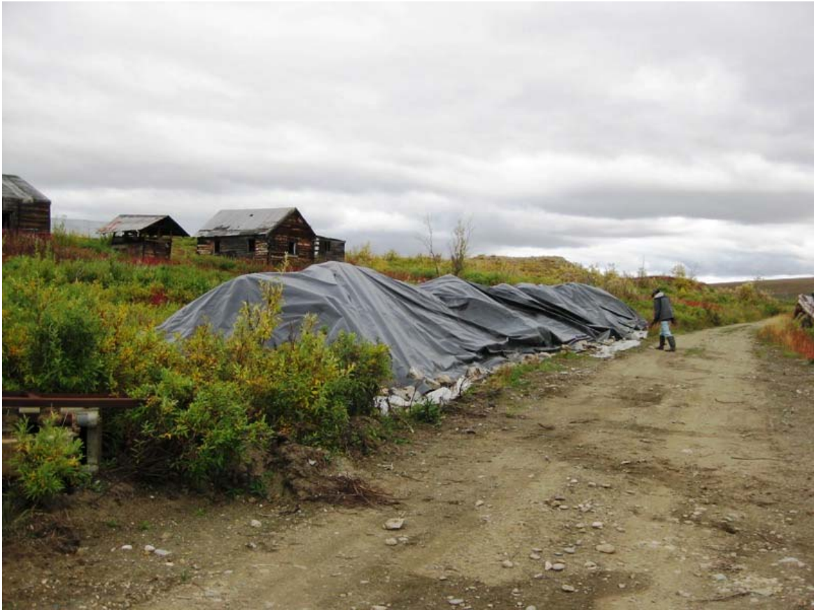
1. Contaminated soil stockpile that was recovered with heavier liner.
