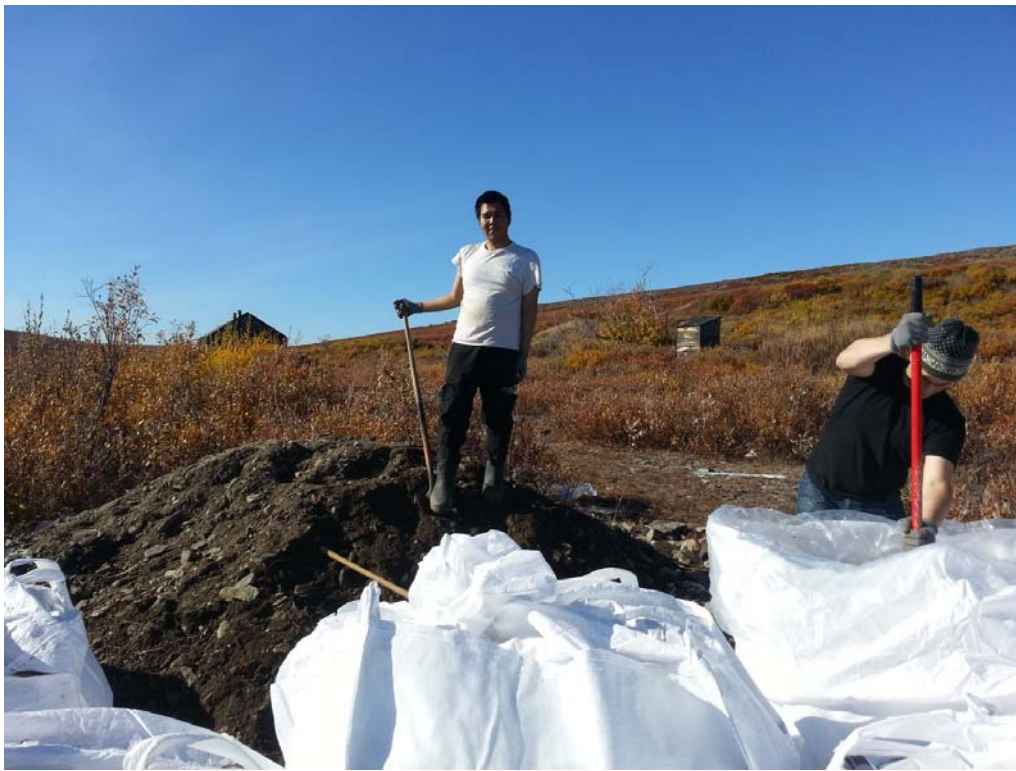
Figure 5: Local hire Clayton Barr and Troy filling supersacks at stockpiles 4 and 5
