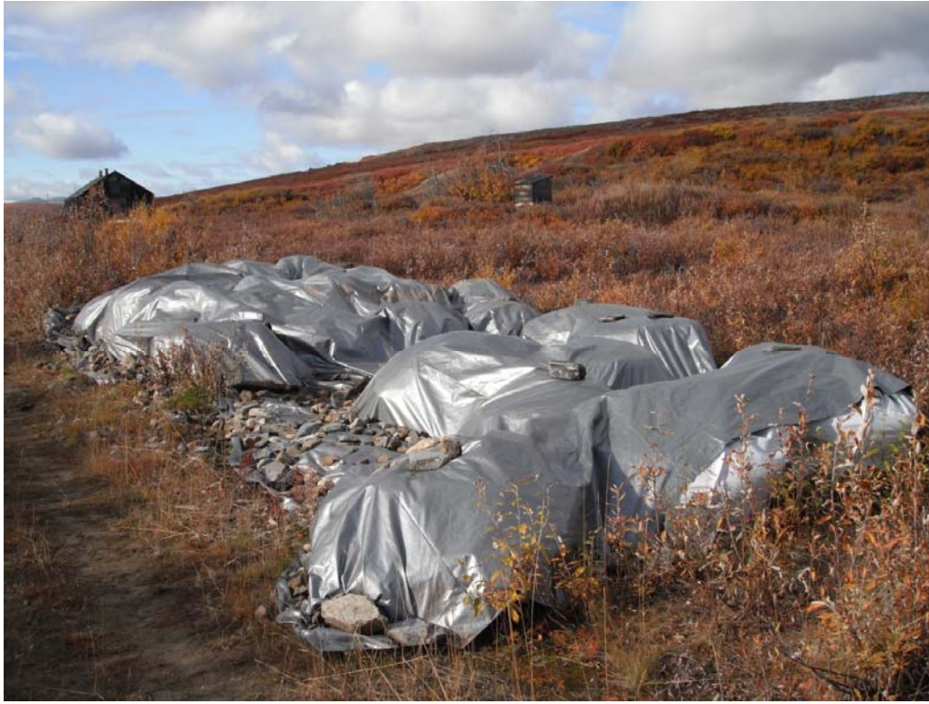
Figure 6: Supersacks filled, covered and awaiting transport
