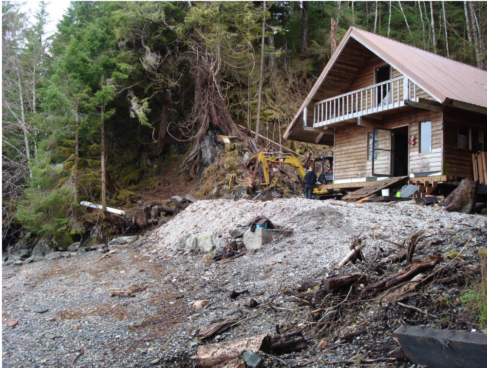
Photo 4: The lodge at Sealevel Mine that was under construction in 2010. The material used as fill is likely mine tailings. Photo courtesy of the State of Alaska Department of Natural Resources.
