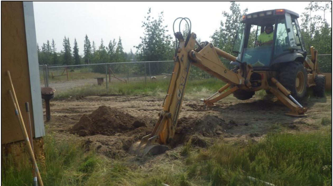
Photograph 8: Excavating Test Pit 2 at Building 100 (facing southeast).
