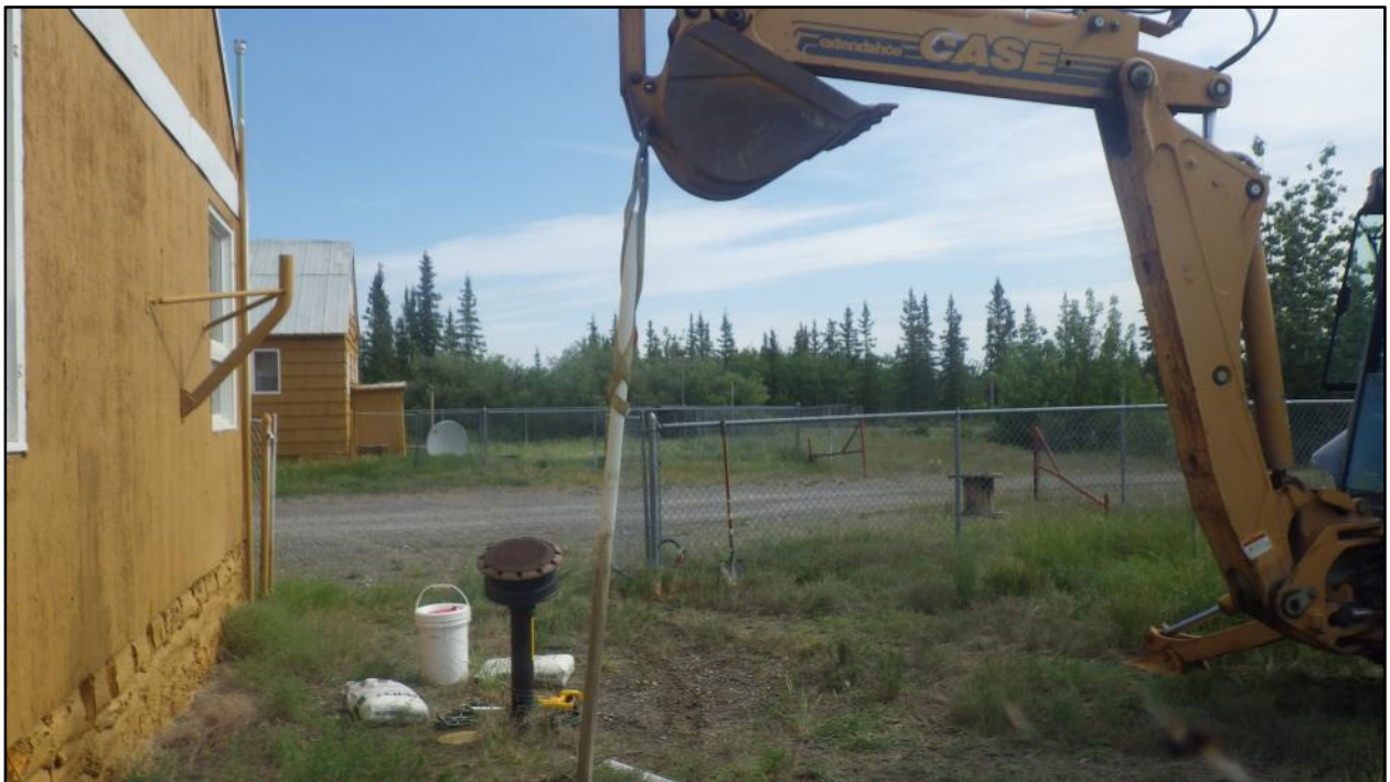
Photograph 2: Removing MW-2 casing at Building 100 (facing east).
