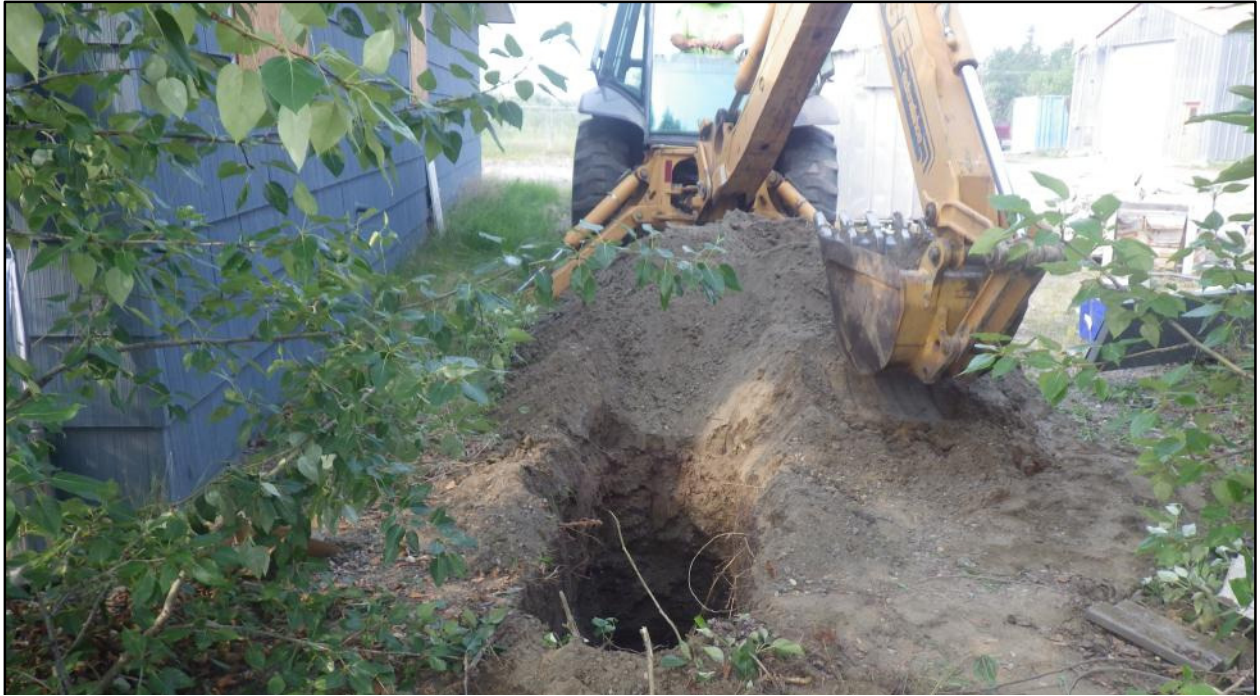
Photograph 7: Excavating Test Pit 2 at the YFHC (facing west).
