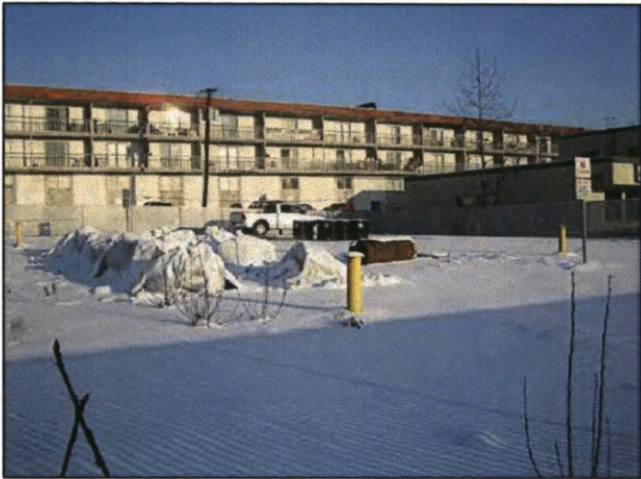
1. Site layout looking Northeast
