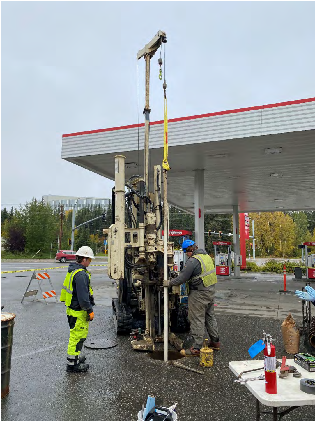
Photo 1: Drillers removing AS-1 to replace with IW-2023-A.
