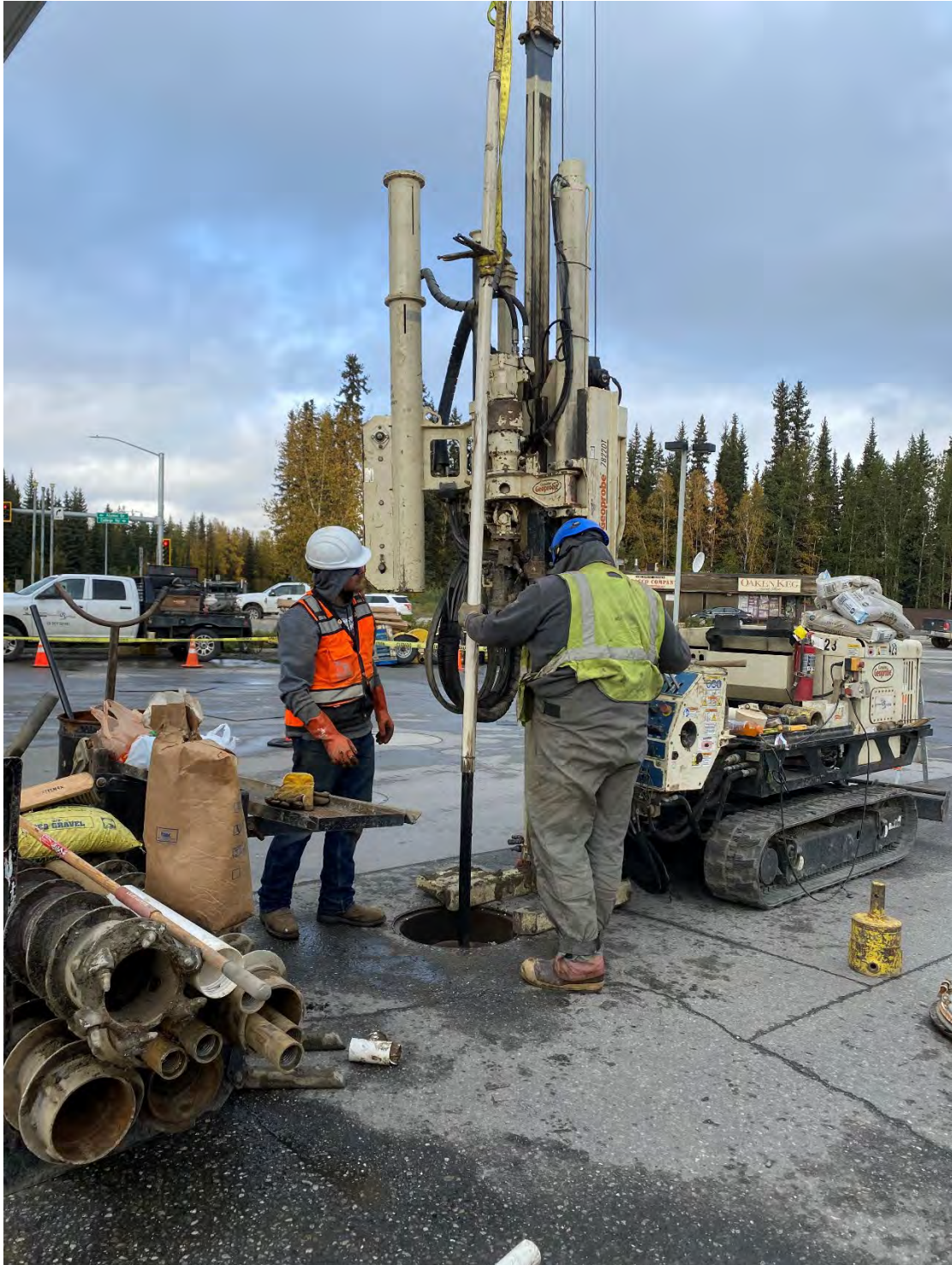
Photo 3: Drillers removing AS-3 to replace with IW-2023-B.
