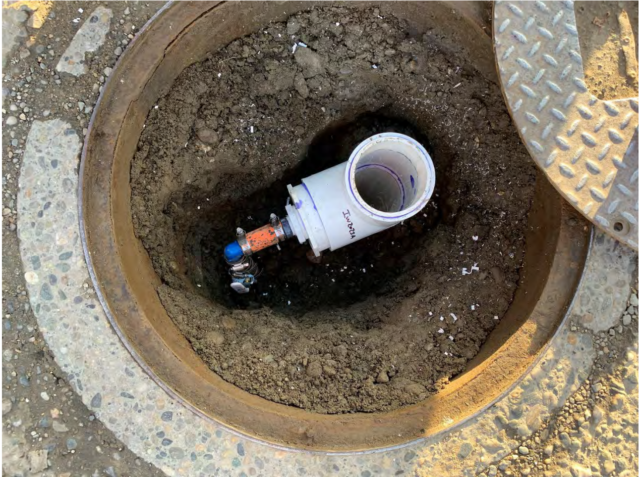
Photo 7: IW-2023-A hooked up to the recirculation system.
