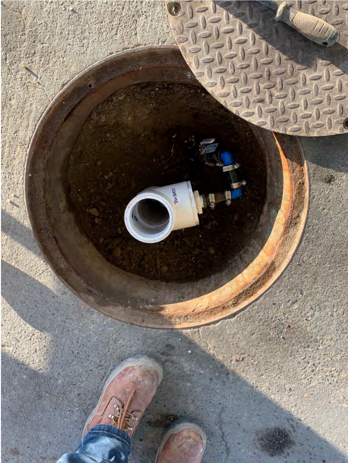
Photo 9: IW-2023-C hooked up to the recirculation system.
