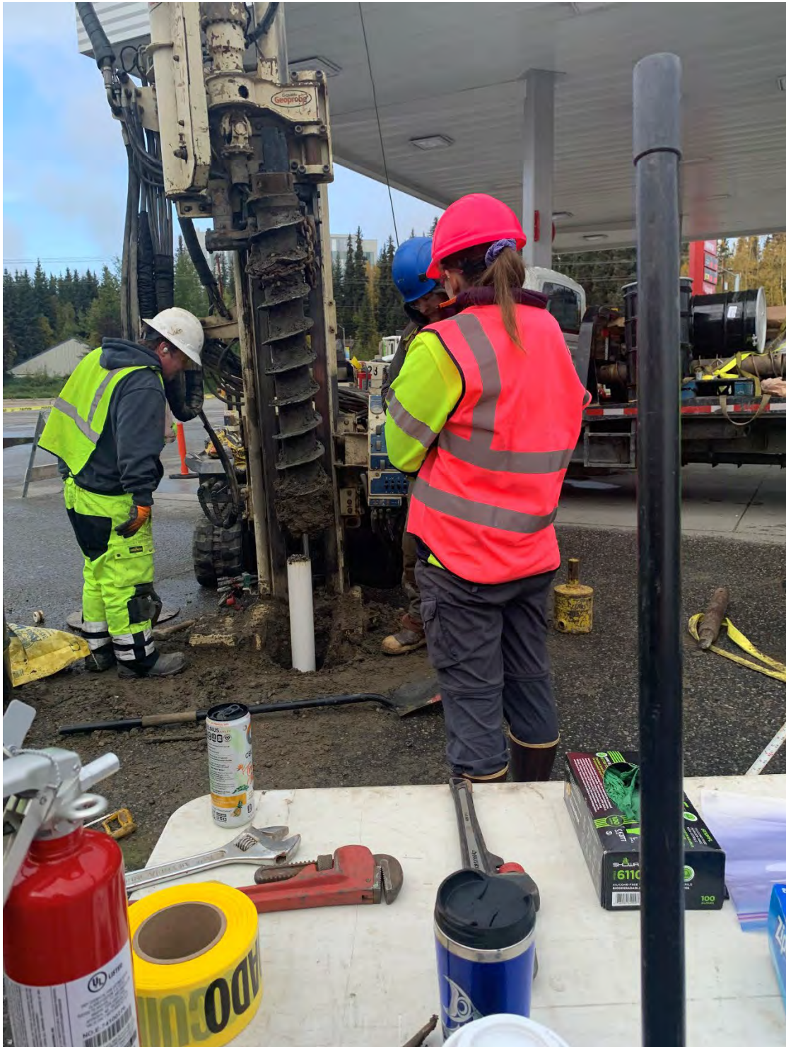
Photo 2: Installing 4" IW-2023-A PVC.
