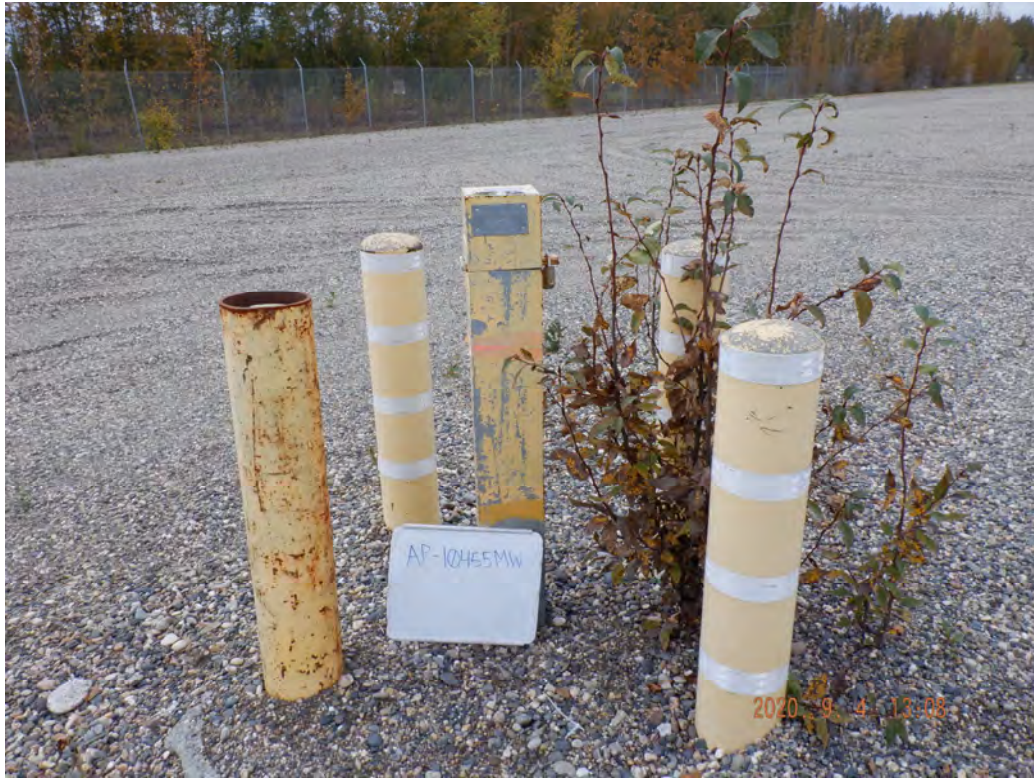
Conducting an IC inspection at OU2; well AP-10445MW is intact and secured (view SW)
