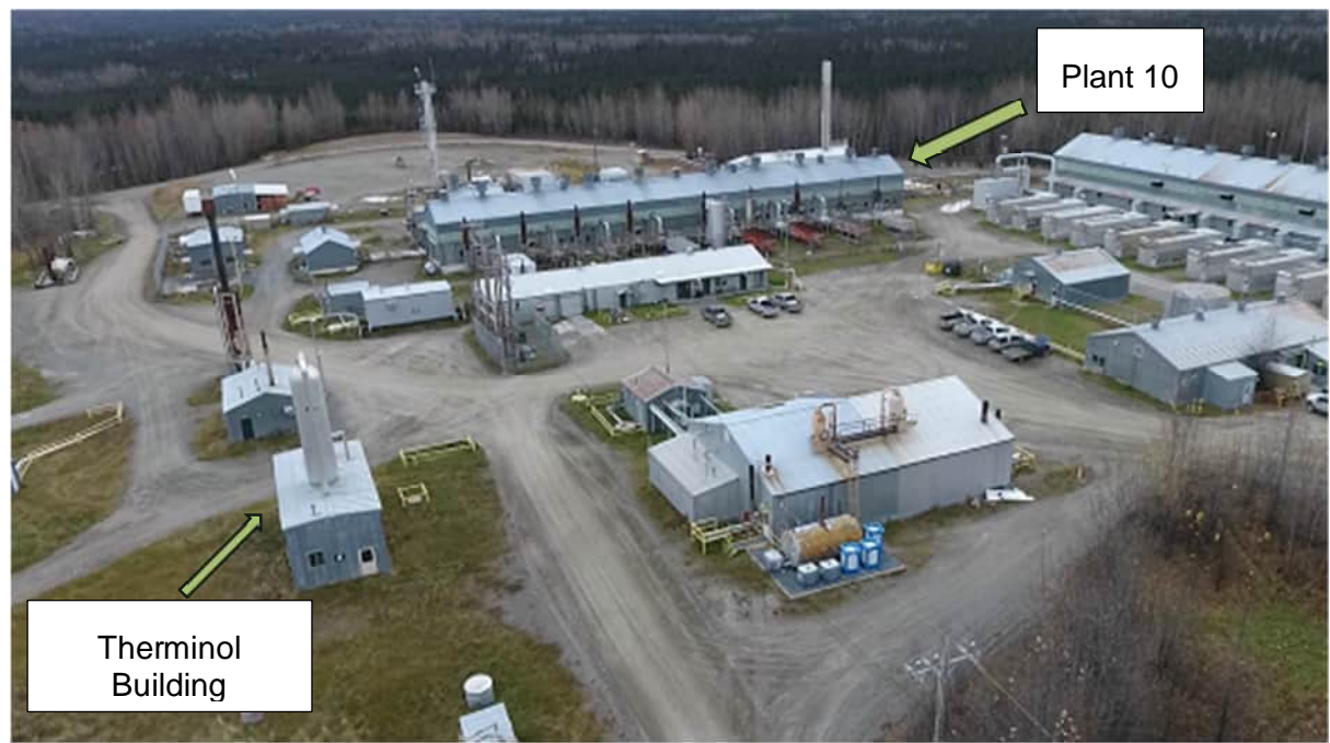
Photo 2: Photo from 2022 showing rebuilt Plant 10. (View From Southwest)
