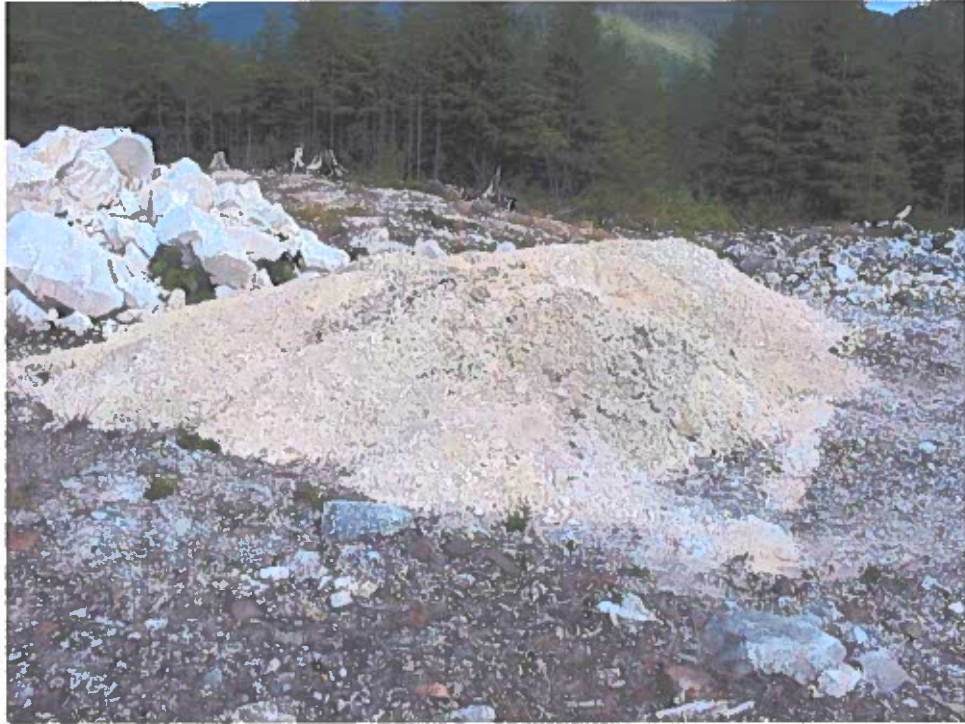
July 31, 2004 Calder Bay Facility, Biocell Site: Fifteen cubic yards of diesel contaminated soil stockpiled on site.
