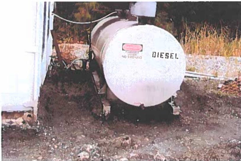
September 2004; Calder Bay Facility, Camp Genset: Close up view showing final depth of excavation of contaminated soil. Contamination left in place beneath fuel tank.
