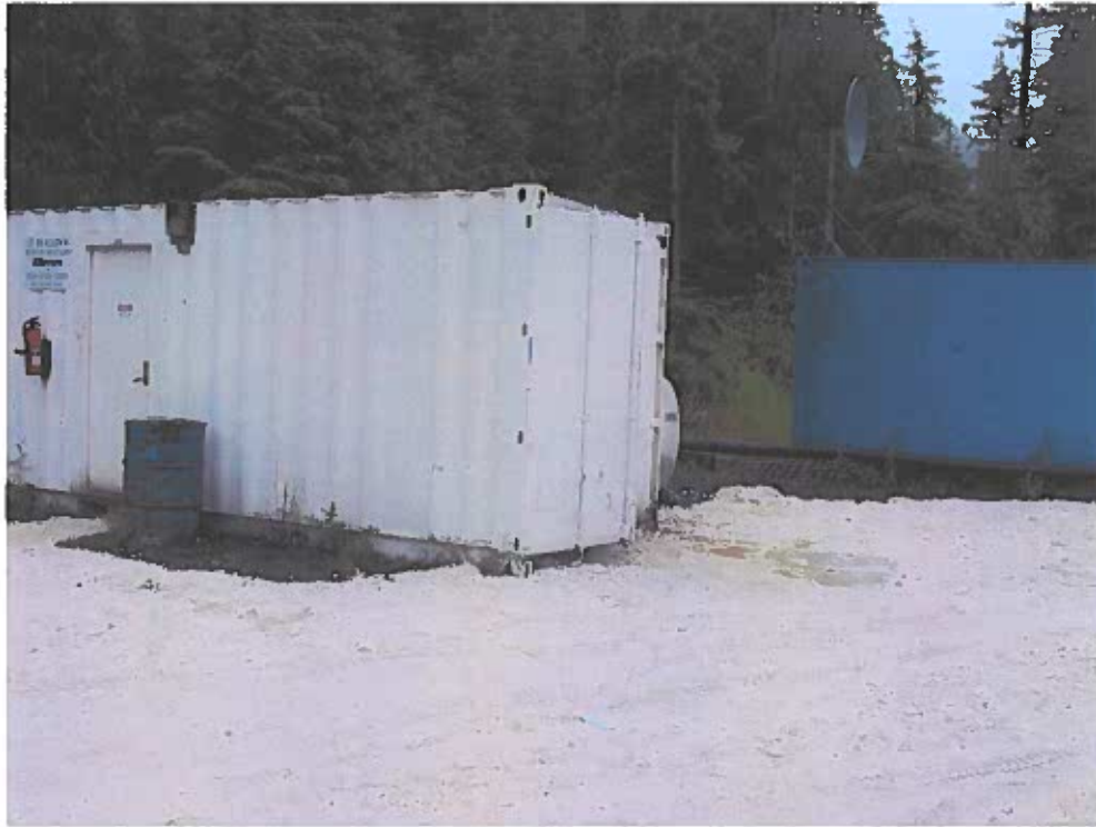
July 31, 2004 Calder Bay Facility, Camp Genset: Light brown stains in calcium carbonate show where petroleum contamination was present.
