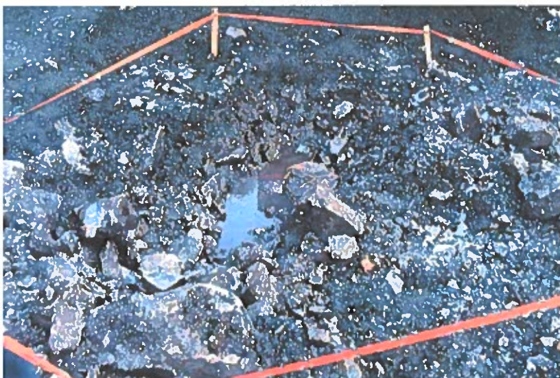
October 9, 2004; Calder Bay Facility, Camp Genset: Close up of Test hole below final excavation, note groundwater.
