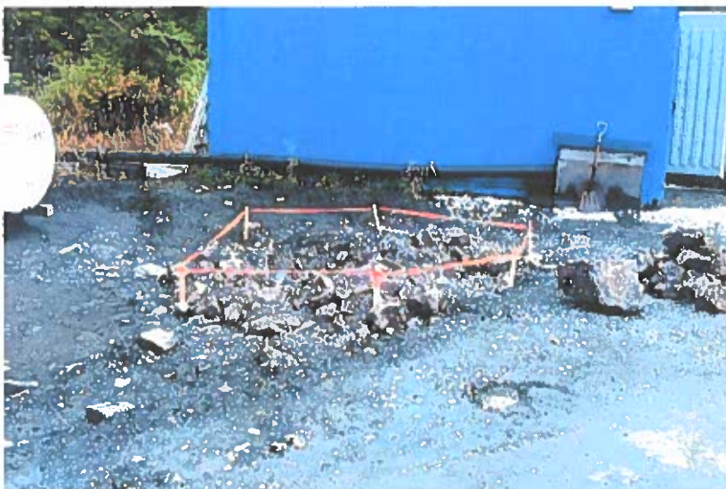
October 9, 2004; Calder Bay Facility, Camp Genset: Test hole below final excavation to find bedrock or groundwater. Final excavation had stopped at shot rock.
