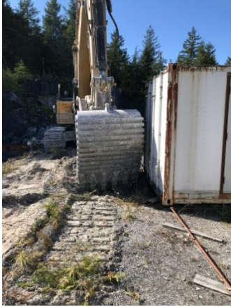
Photo #7 CS8 Sample Location
