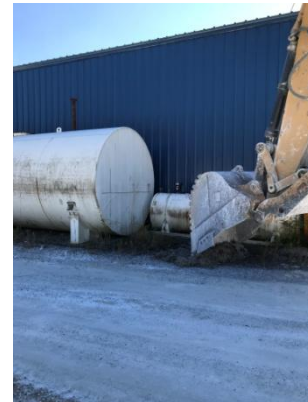
Photo #10 CS12 Sample Location
