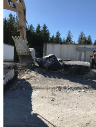
Photo #8 CS7 Sample Location
